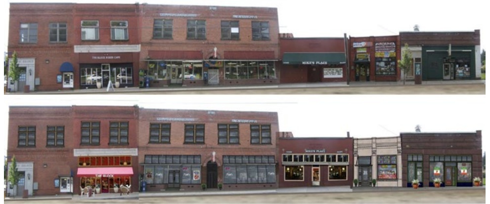
(Top) Dayton downtown block before restoration. (Bottom) Dayton downtown block design assistance suggestions, including revealing covered transom windows.
