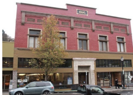
Oregon City's Busch Building before project started (top). Busch Building during construction (middle). Busch Building after project is completed (bottom).
