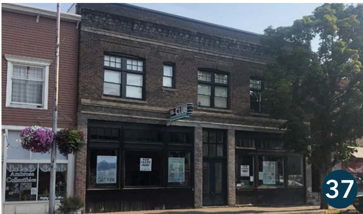
ADDRESS: 522 EAST MAIN DATE OF CONSTRUCTION: 1907 HISTORIC NAME: THE STEWART AND PORTER BUILDING
