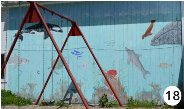
NAME: UNDERWATER WORLD * ADDRESS: 403 NORTH RIVER ROAD CONDITION: FAIR RISK LEVEL: HIGH
