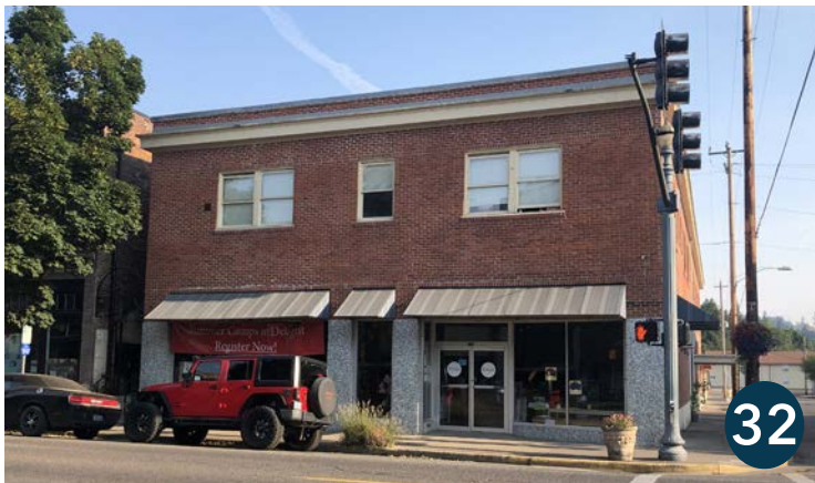
ADDRESS: 17 N 6TH DATE OF CONSTRUCTION: 1923 HISTORIC NAME: OMER APARTMENTS/ KERN BUILDING
