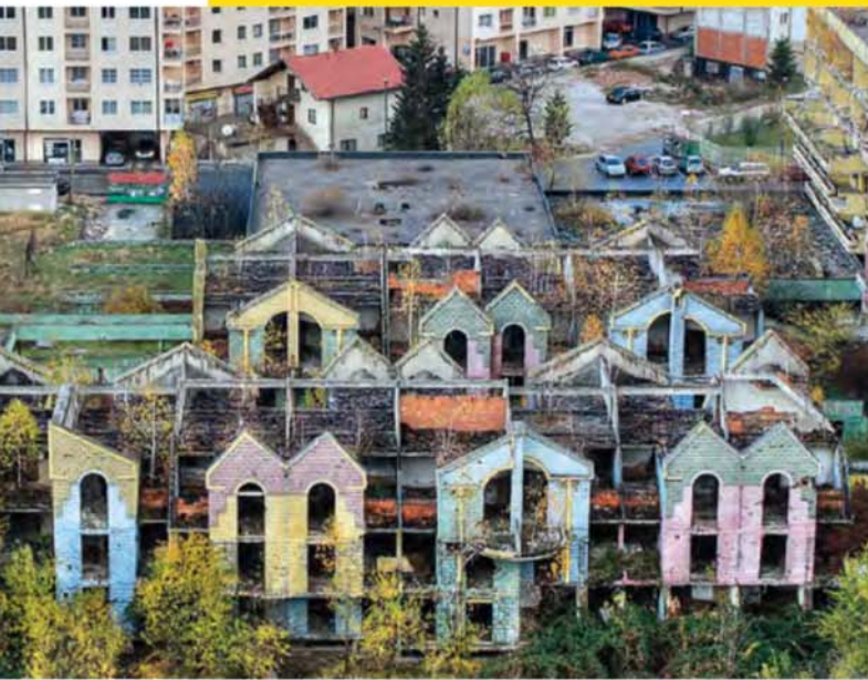
Building destroyed during the 1992–1995 civil war, Sarajevo, Bosnia and Herzegovina. © akturer / Shutterstock.com*
