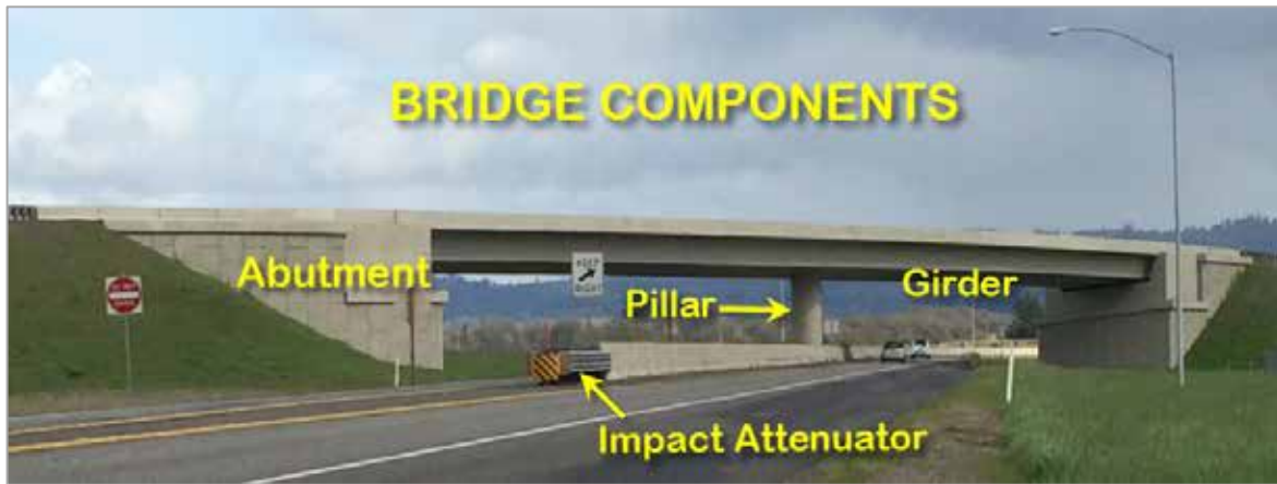
Figure 64. Bridge Components
