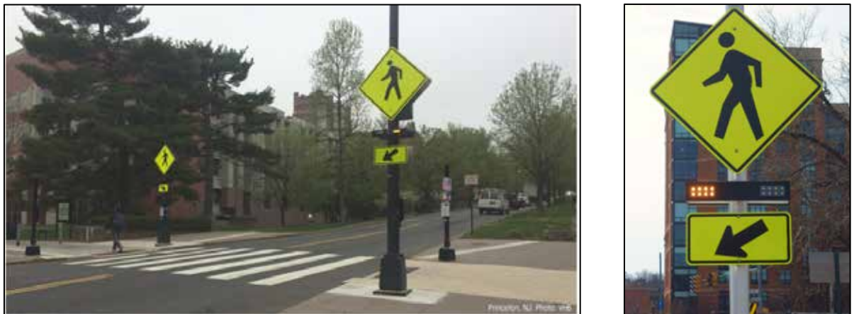
Figure 59. Pedestrian Signal - Rectangular Rapid-Flashing Beacon (RRFB)
