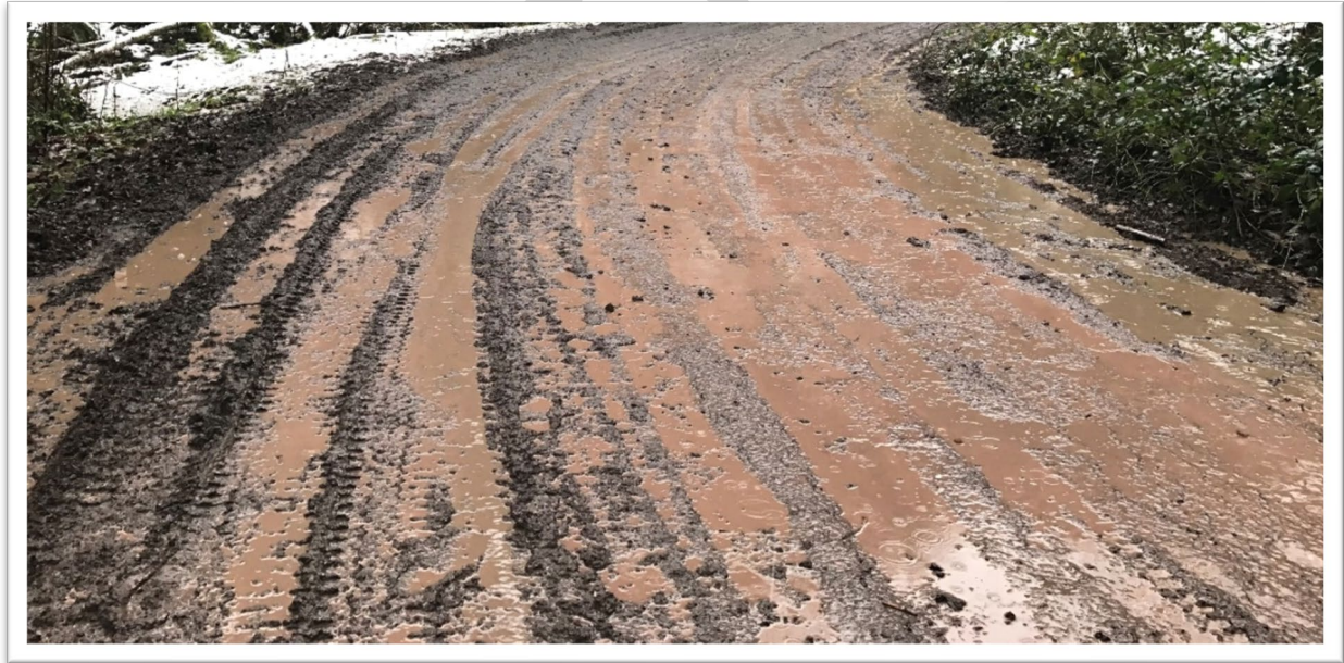
Photo 5. Road surface with a layer of mud and rutting [recommend using a different image].
