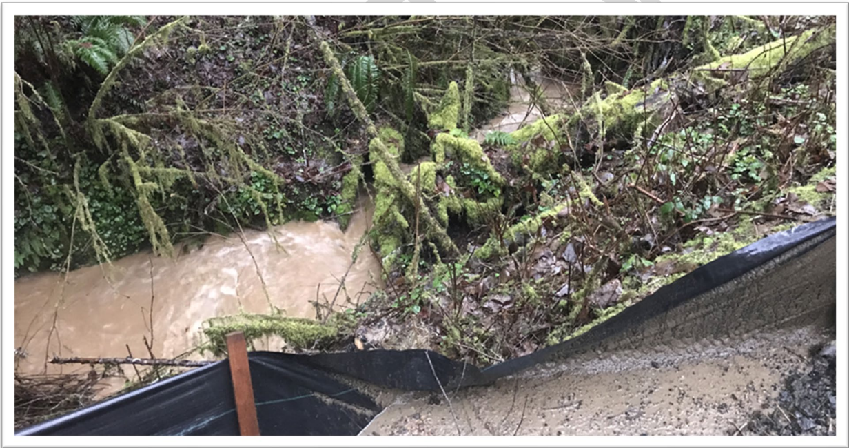
Photo 2. Example of other measure, sediment trapping using silt fencing.
