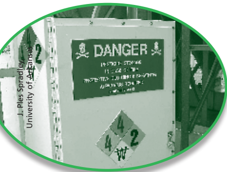
A National Fire Protection Association (NFPA) warning on a storage box for fumigants. The strikeover on the letter W in the white diamond alerts firefighters not to use water to put out a fire.
