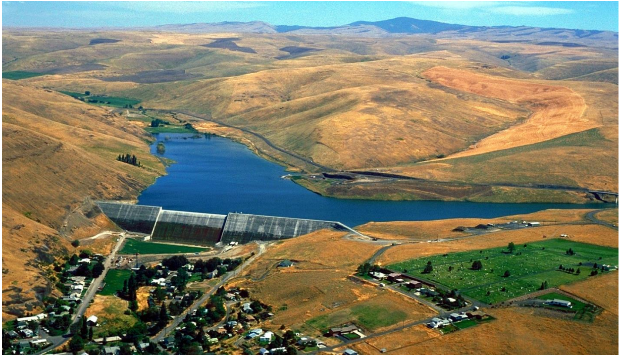
Willow Creek Dam above the City of Heppner
