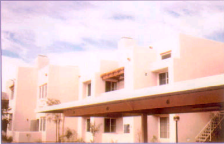
Two story multi-family complex with Type V construction. (CS3-1)
