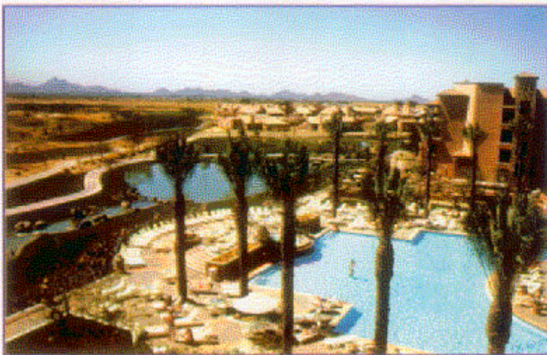
An overall view of the resort and the direct connection to the Tournament Players Club. The requirements for 360 degree access was modified due to complete automatic sprinkler protection. (CS 1-2)
