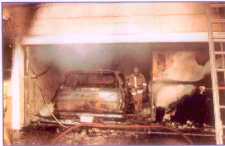
The results of a typical garage fire. (CS5-1)
