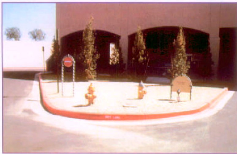
Two hydrants near the access to the underground parking. One hydrant uses grey water and the other is connected to an 8" domestic supply. (CS1-4)
