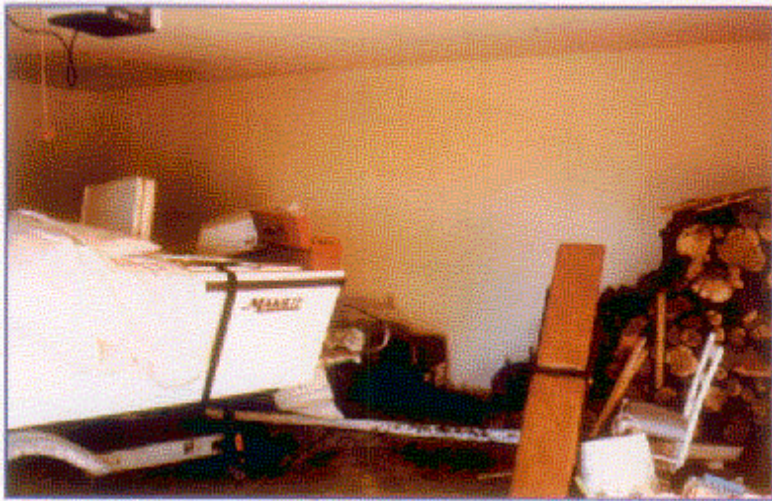
The fire started from ashes in a paper bag placed next to combustible materials (CS4-2)
