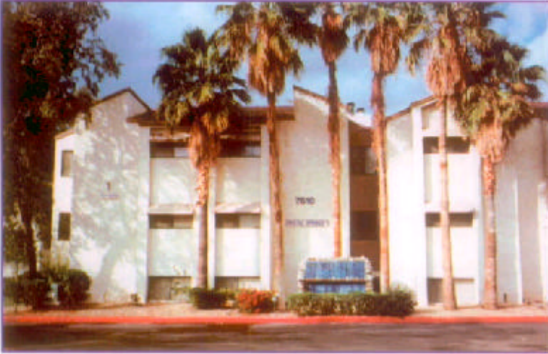
Typical three story multi-family complex of Type V construction. (CS2-1)
