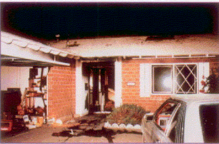
A closeup view of the structure the evening of the fire. Upon arrival fire crews had flames rolling out of the front door over their heads and the dispatch center had not yet received a 911 call from the public. (CS9-2)
