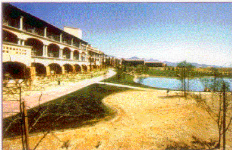
The Scottsdale Princess Resort uses this 2.5 million gallon grey water feature and a 2,000 (CS1-1) fire pump to provide the initial supply for the automatic sprinkler system. (CS 1-3)
