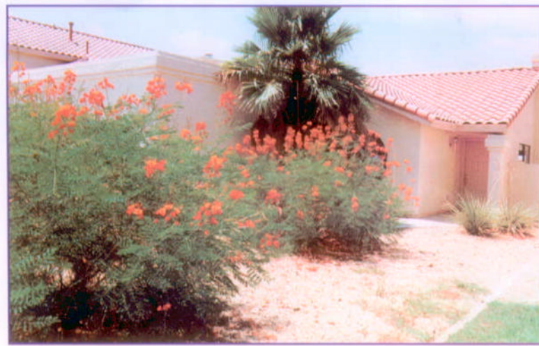
A typical suburban Scottsdale home consisting of lightweight construction and a heavy tile roof. (CS6-1)
