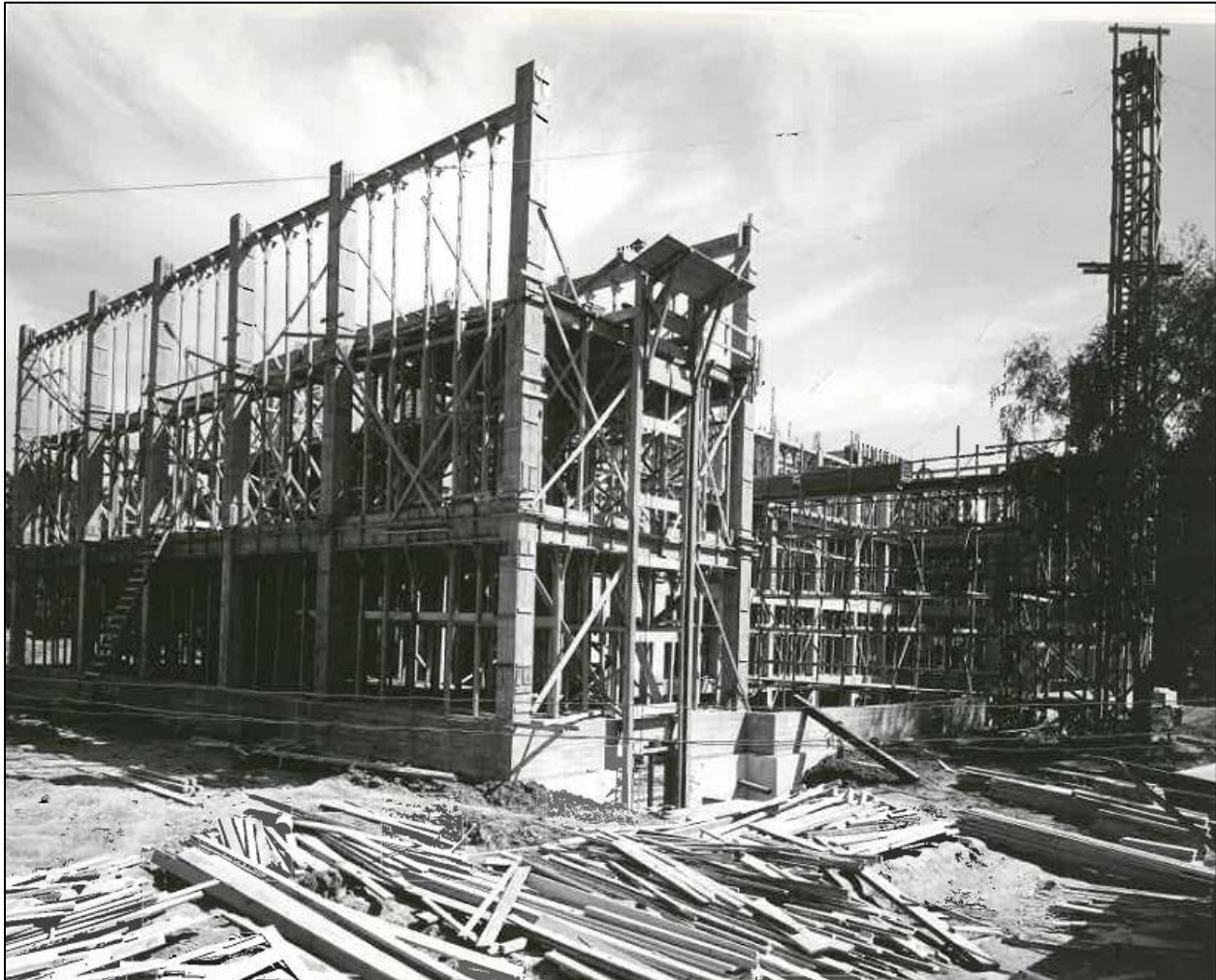
Figure 16 – Construction of State Library June 1, 1938, from northeast side.
