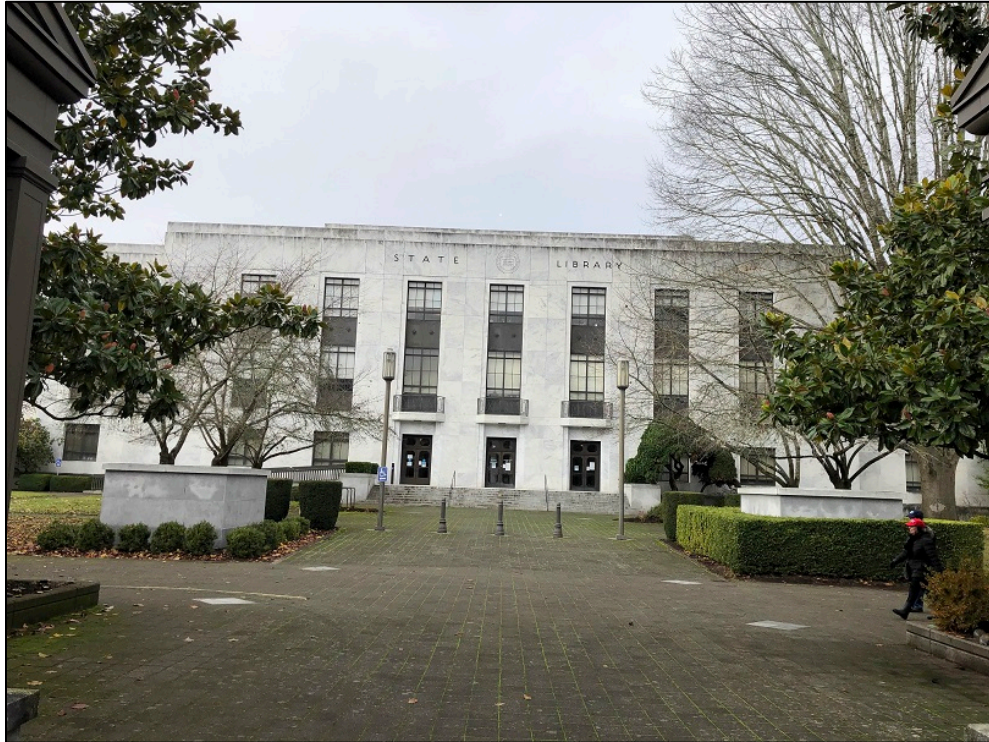
Photo 1 of 15 – OR_MarionCounty_StateLibrary_0001; State Library and setting, facing west
