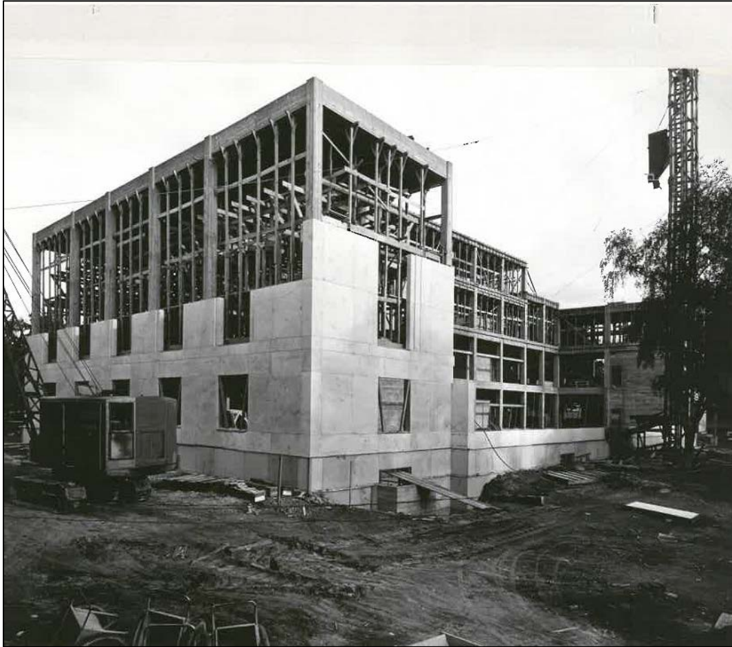
Figure 17 – Construction of State Library building, July 2, 1938, from northwest side.
