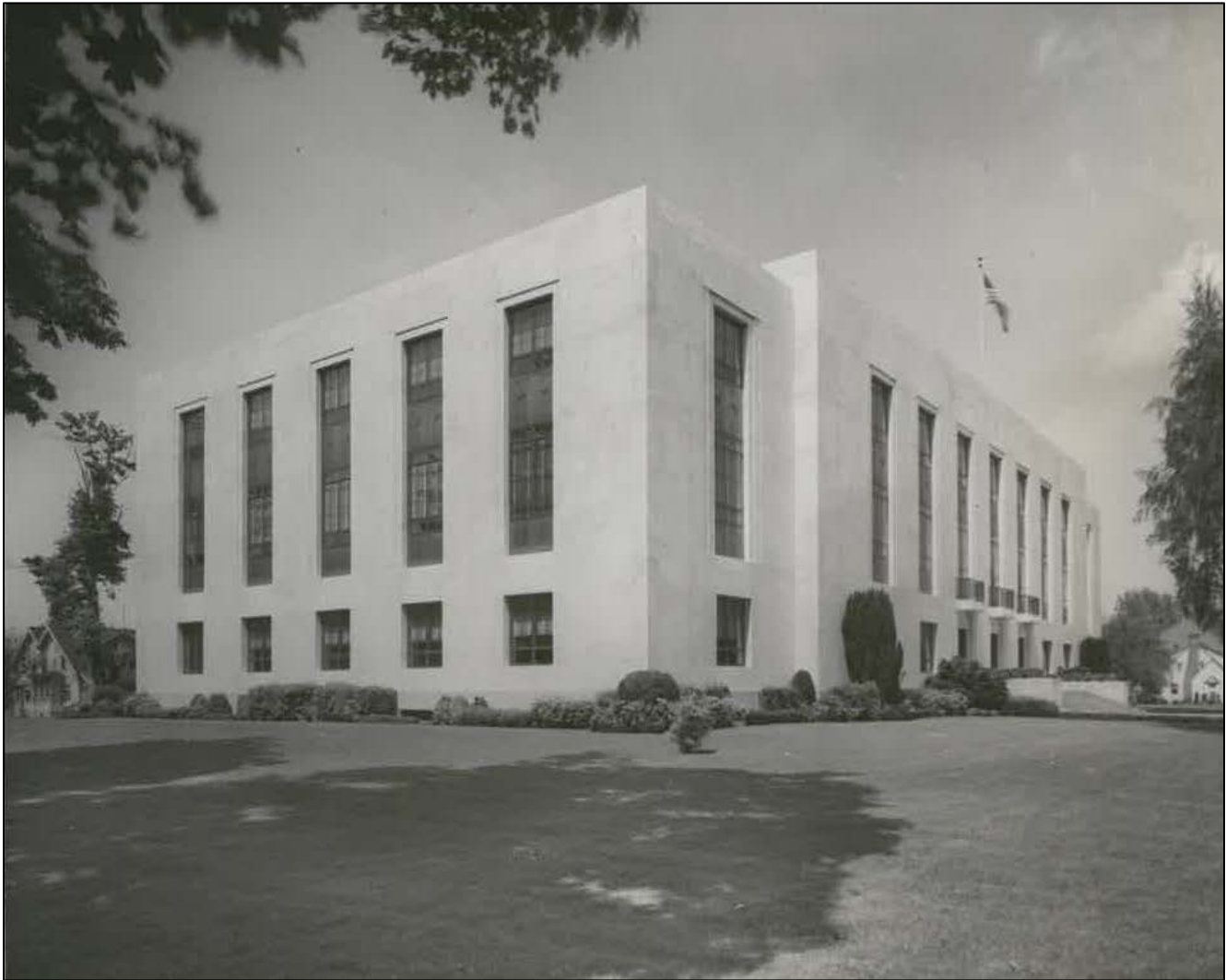
Figure 20 – Exterior of completed building from southeast corner, c. February 1939, Boychuk Studio photographers.
