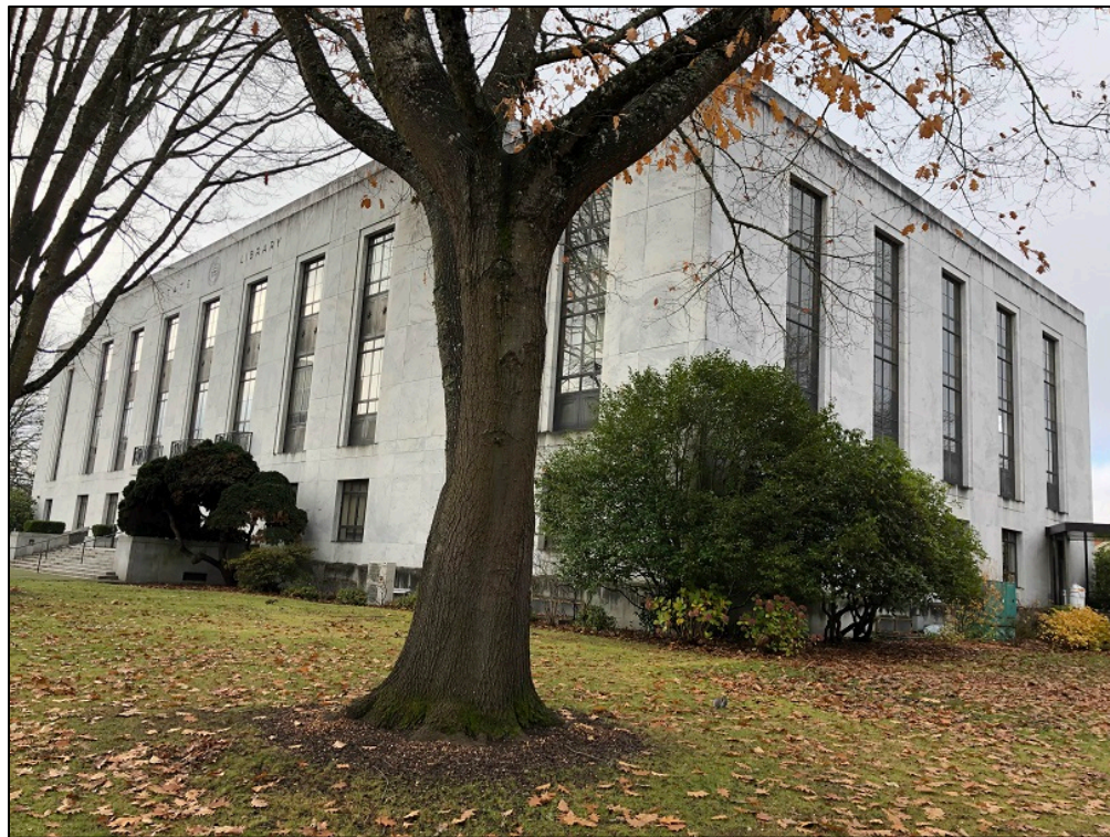
Photo 2 of 15 - OR_MarionCounty_StateLibrary_0002; State Library northeast corner of building, facing southwest
