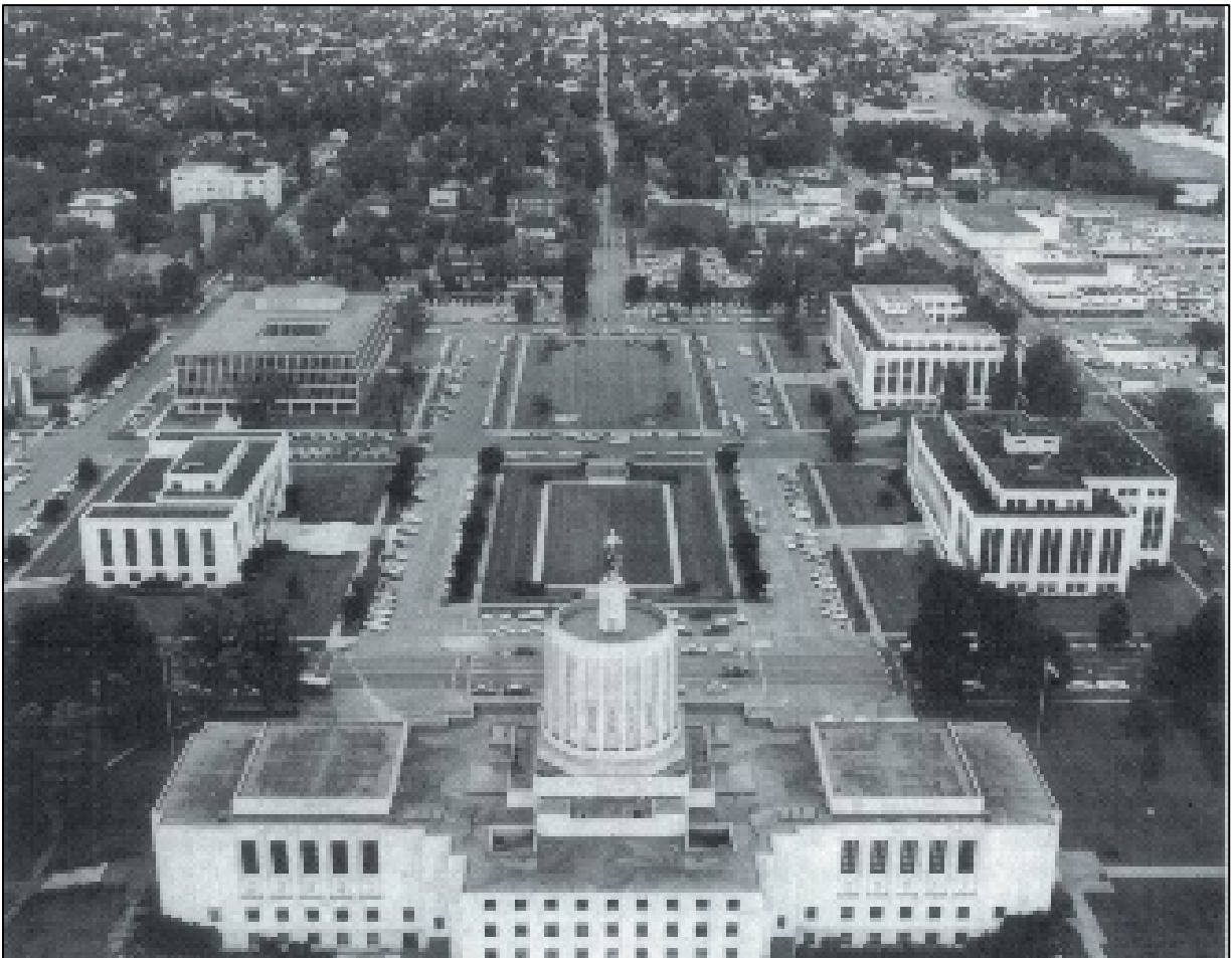
Figure 10 - This historic photograph shows the setting of the State Library in relation to the State Capitol, the Capitol Mall, and adjacent state administrative offices in 1962, facing north. (3 of 53/ODOT K7012, in National Register Registration form for Oregon State Capitol)
