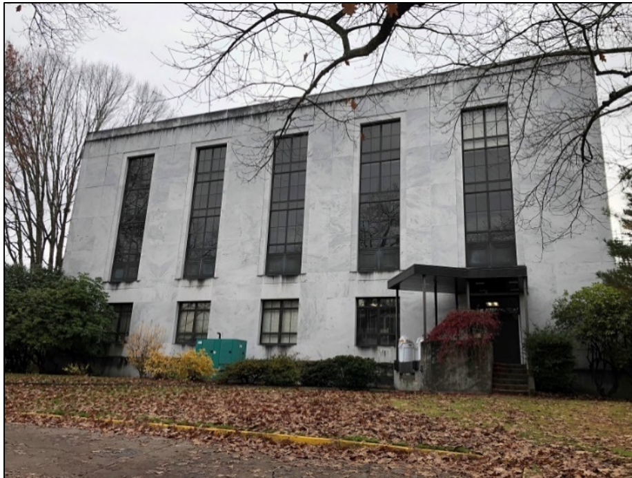
Photo 7 of 15 - OR_MarionCounty_StateLibrary_0007; State Library north side, loading dock on west corner result of alteration, landscaping includes several trees identified on the State Capitol State Park walking tour: Dove Tree ( Davidia involucrata ) and Northern Red Oak ( Quercus rubra ), facing south
