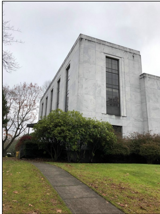
Photo 3 of 15 - OR_MarionCounty_StateLibrary_0003; state library southwest corner of building, facing northeast
