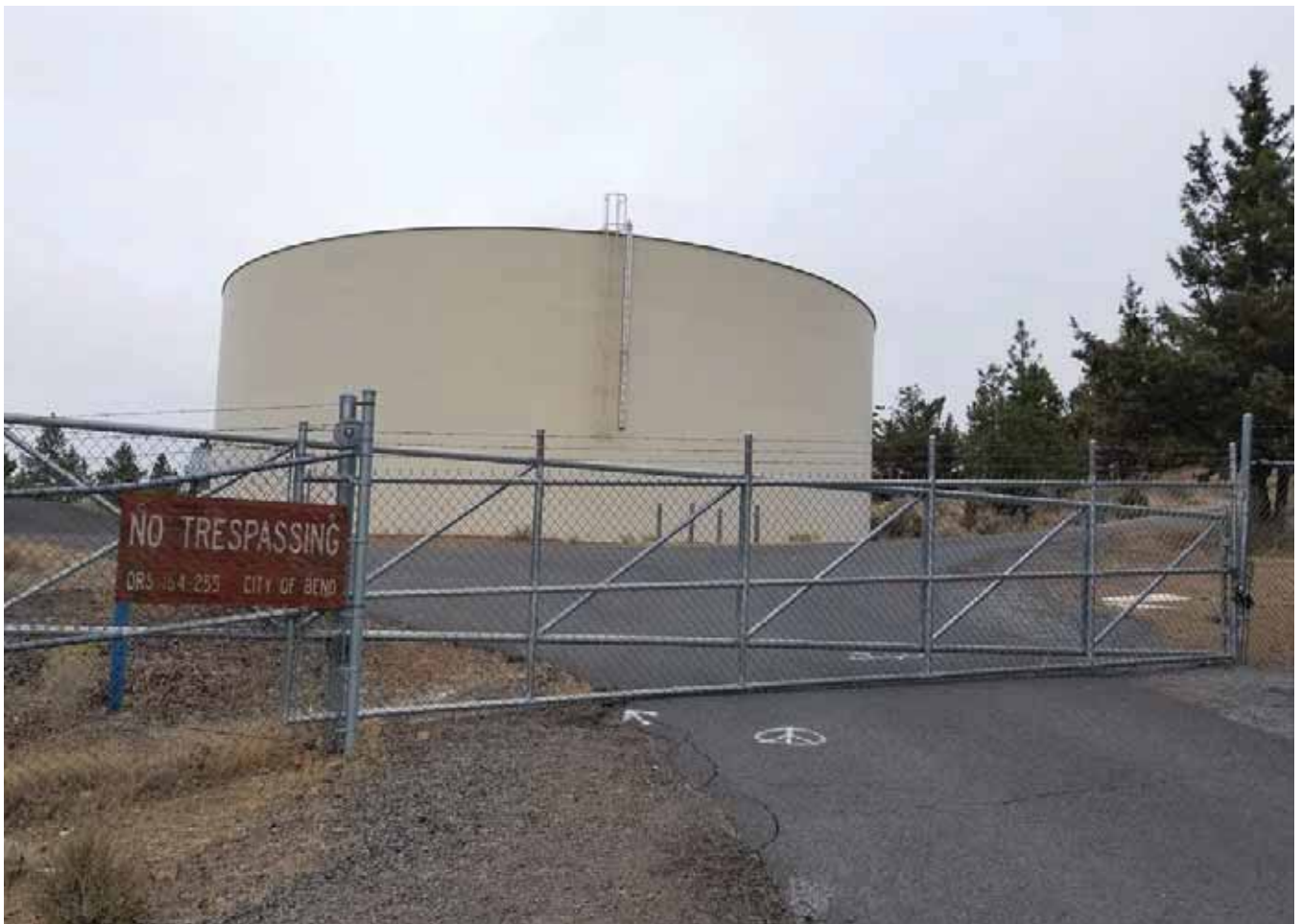
City of Bend water facility on north boundary of the park.
