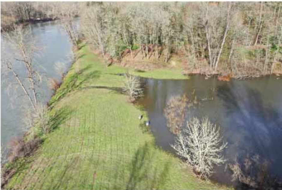
The pond behind the revetment empties into the Willamette River.
