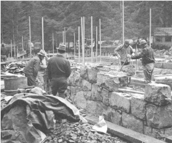
Foundational stonework for today's South Falls Lodge at Silver Falls.
