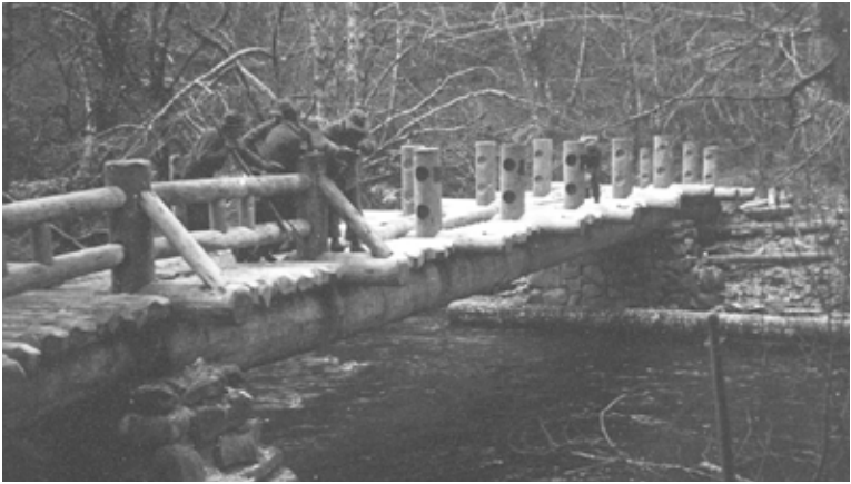
Building a footbridge in Silver Falls State Park.
