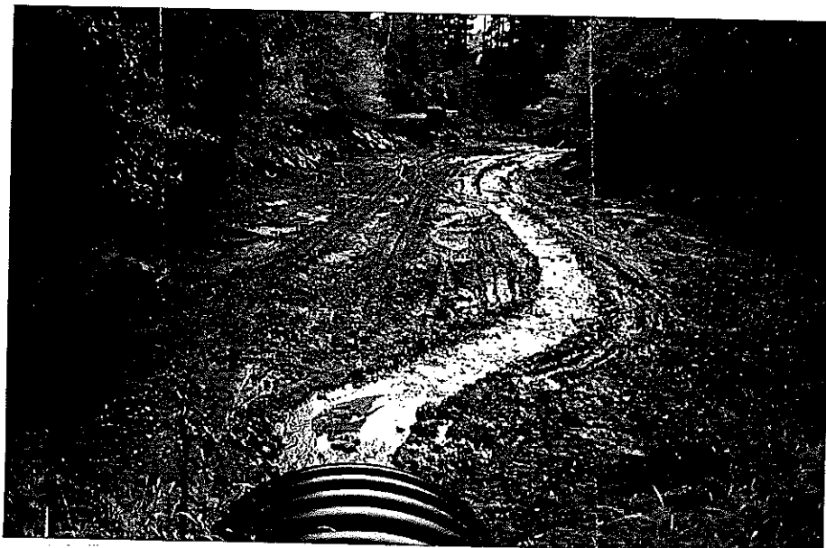
The North Depoe Bay Creek runs through the city's drained water reservoir during renovations to the site on Monday, Sept. 19. Water plant operators drained the reservoir in July to remove 6,000 cubic yards of silt and rebuild access platforms. (Photos by Nathan Howard)
