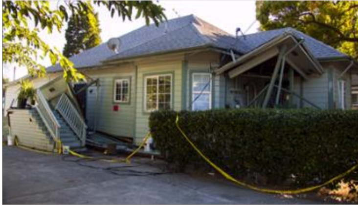
Crawlspace (Cripple wall)
