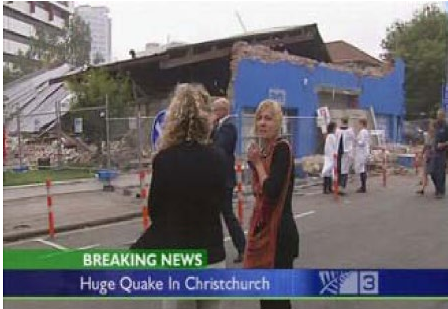
132 Kilmore St. URM damaged in Sept Earthquake After 2-22
