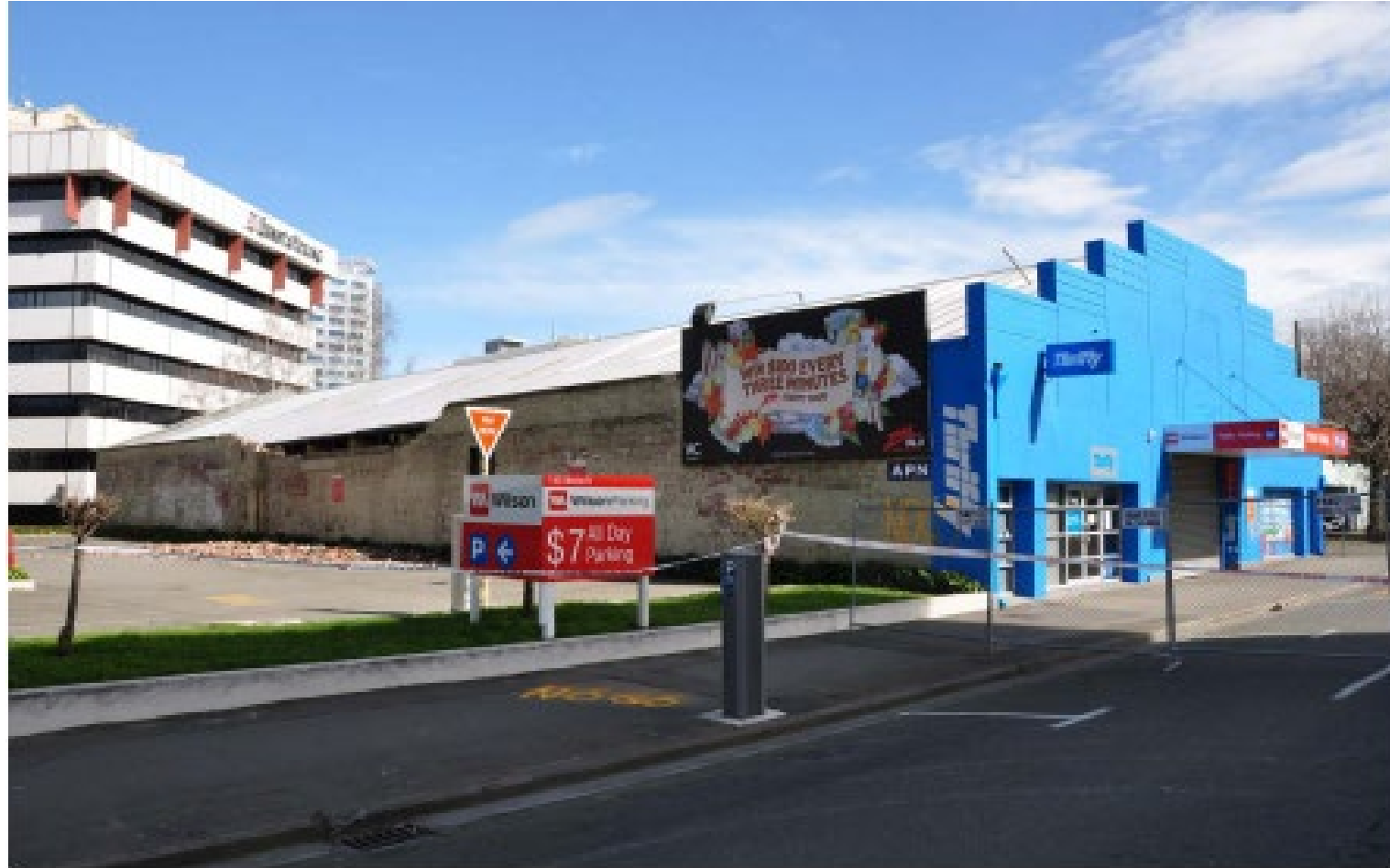
132 Kilmore St. URM damaged in Sept Earthquake Before 2-22
