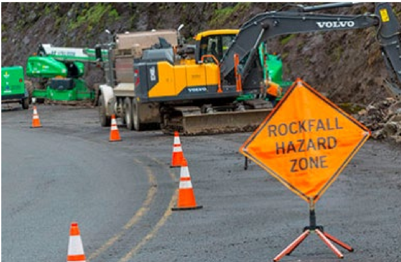
6-6 Repairing Slopes along Oregon 244 to prevent rock fall.
