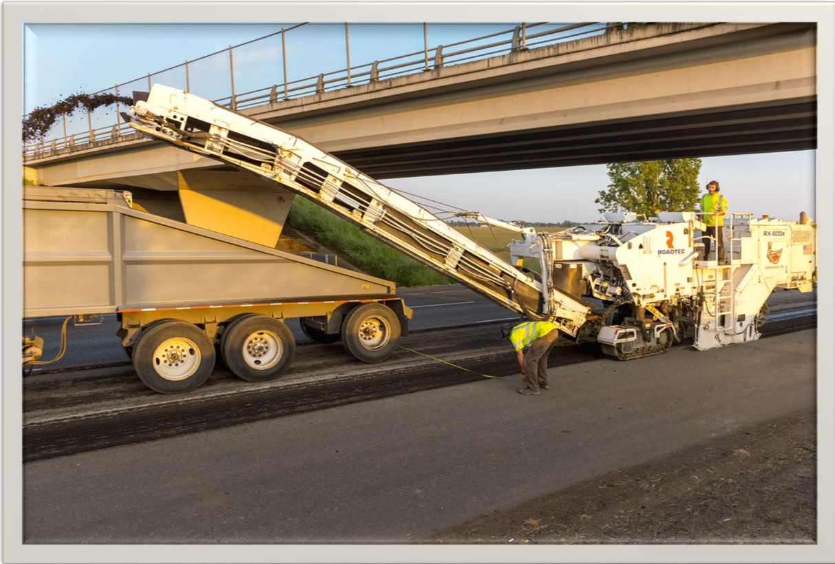
Interstate 5 Paving from Woodburn to Salem, May 2019
