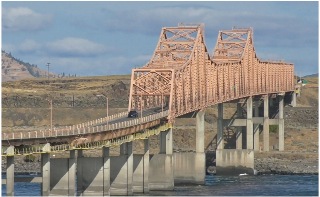
2-3 The Dalles Bridge, The Dalles, Oregon
