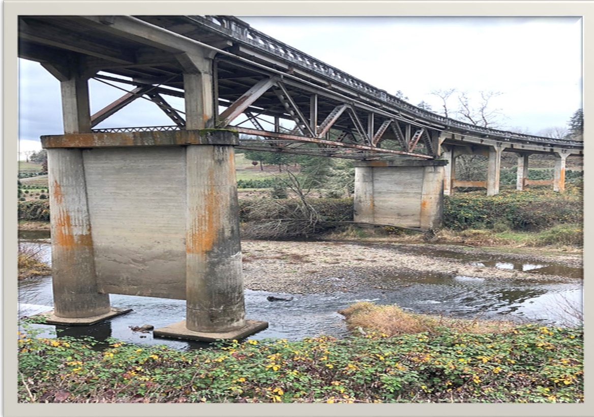
Oakland Bridge Piers
