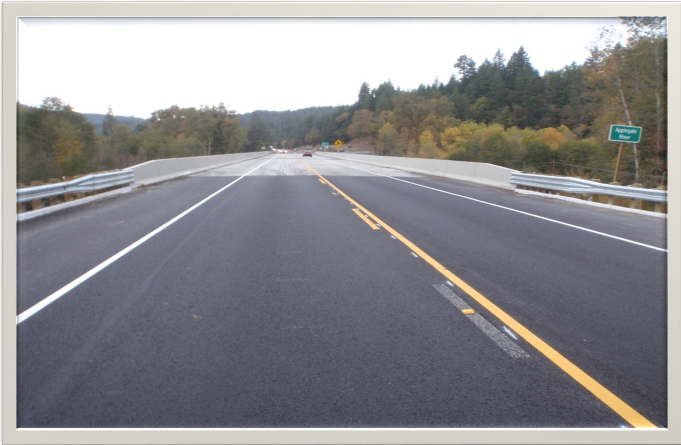
U.S. 199, Applegate River Bridge, SW of Grants Pass
