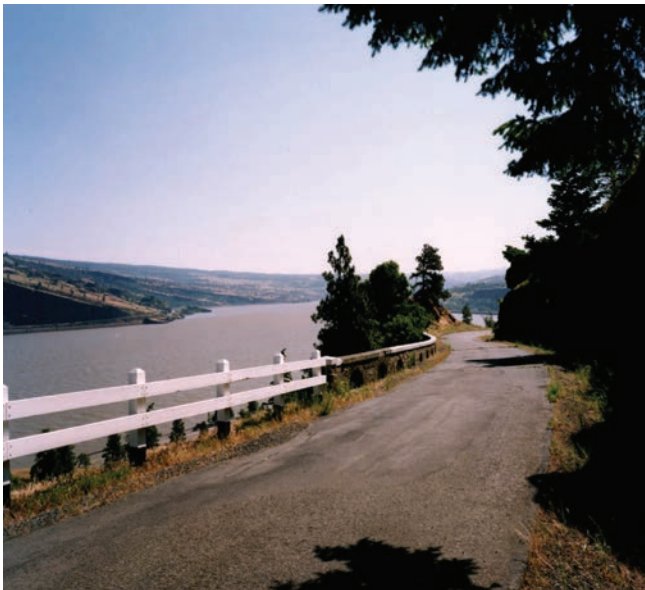
Figure 34—Restored Rubble Masonry Parapet Wall and Guardrail
