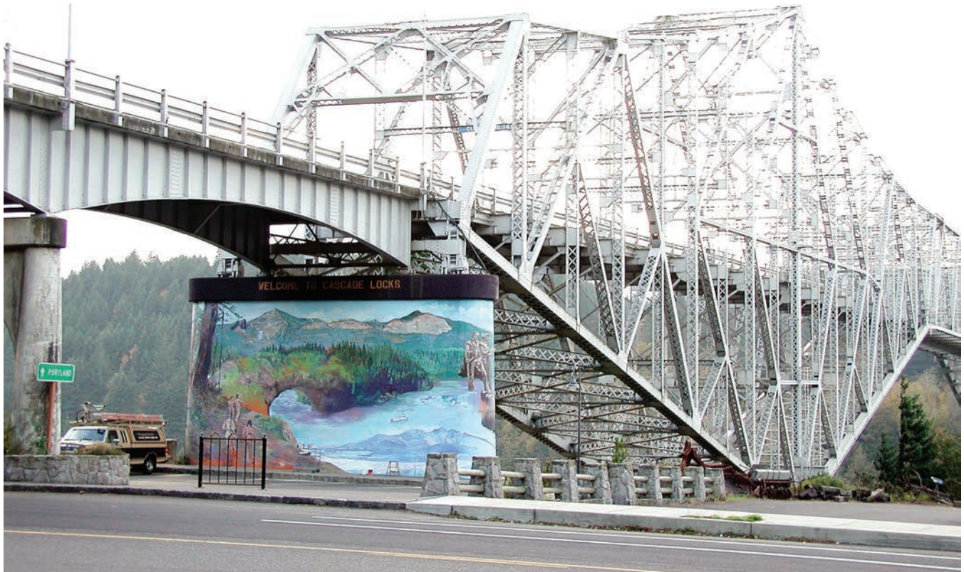
Figure 26—Bridge of the Gods featuring the Cascade Locks Mural
