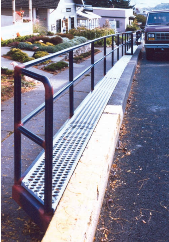
Figure 31—Pedestrian Railing in Hood River
