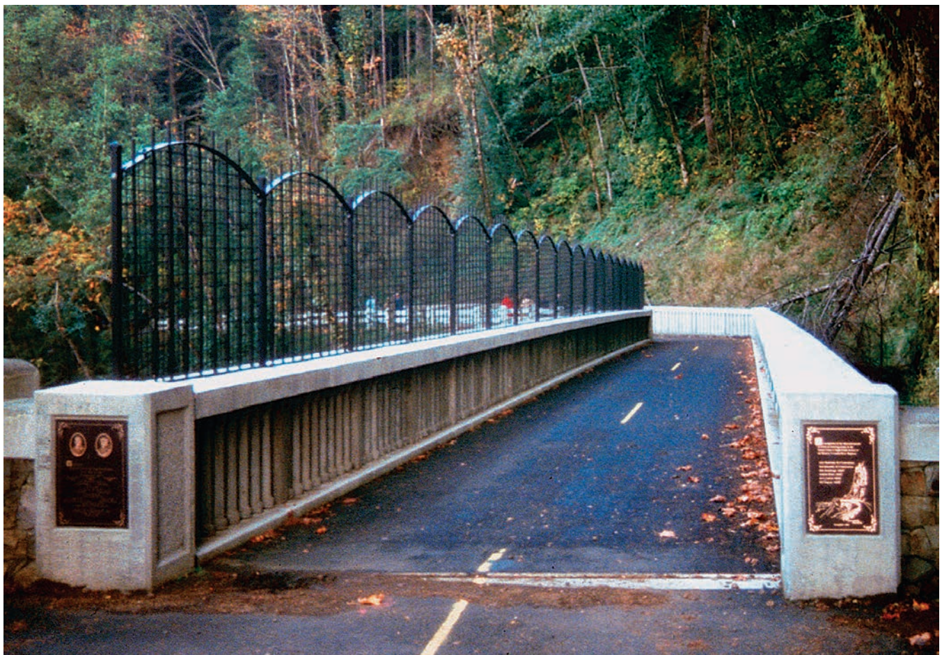
Figure 23—Toothrock Tunnel Bridge
