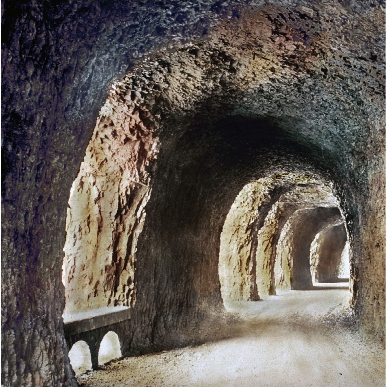
Figure 28—Mitchell Point Tunnel—The Tunnel of Many Vistas
