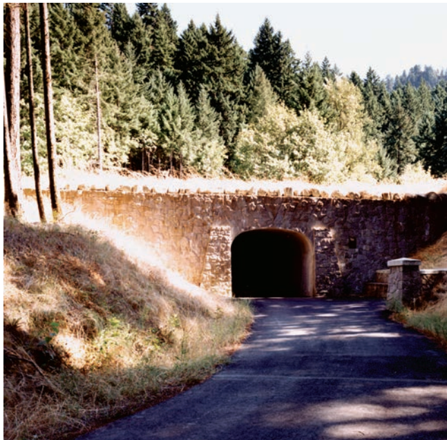
Figure 25—HCRH State Trail Undercrossing Interstate 84 Between Eagle Creek and Cascade Locks
