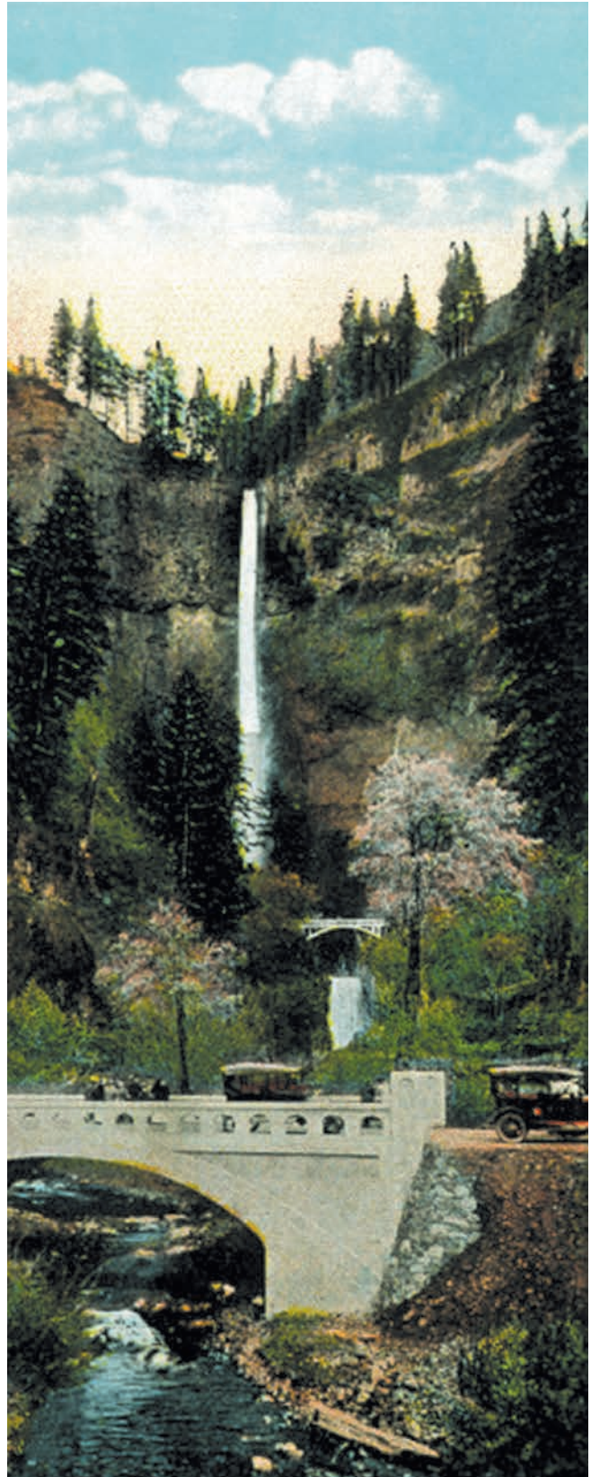
Figure 16—Multnomah Falls, Benson Footbridge and Multnomah Creek Bridge
