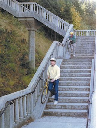
Figure 83—Groove included on Stairway allows for Bike Access
