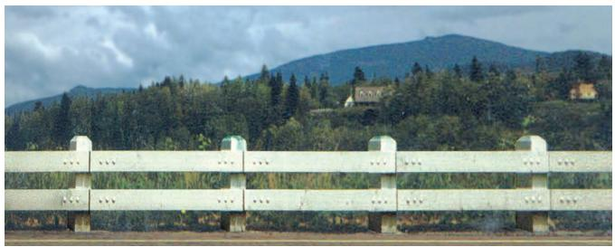
Figure 61—Two-Rail, Steel-Backed, Wooden Guardrail
