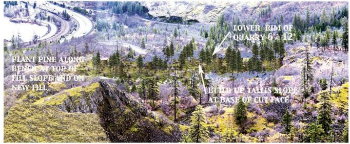
Figure 75—Simulation of Restoration of Rowena Pit
