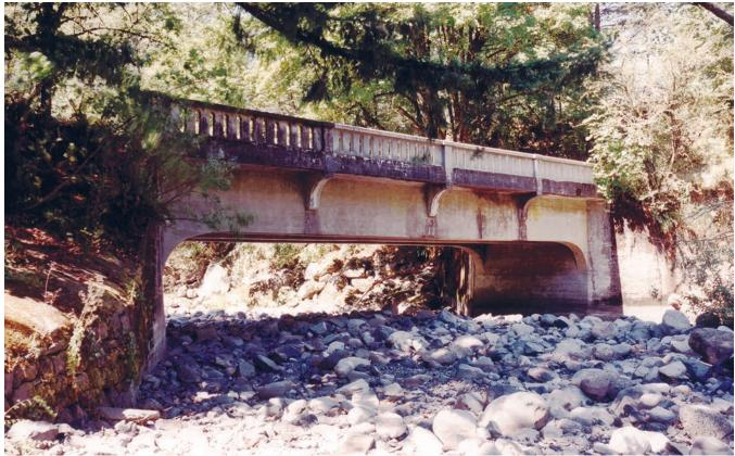
Figure 102—Tanner Creek Bridge Railing Repaired
