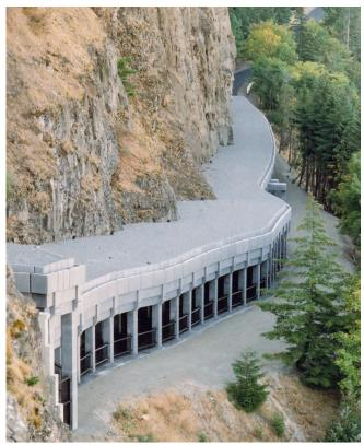
Figure 89—Rockfall Catchment from Above
