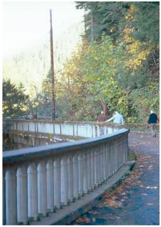
Figure 78—Toothrock Viaduct Railing Repaired
