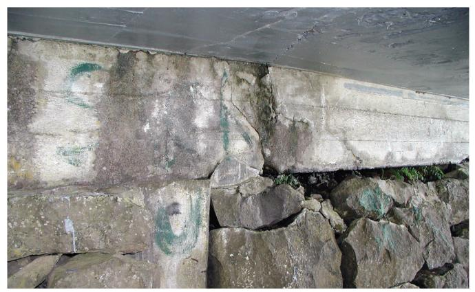
Figure 77—Deterioration of the Crown Point Viaduct
