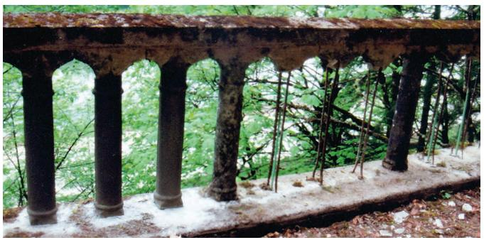
Figure 79—Toothrock Viaduct Railing deteriorated Condition
