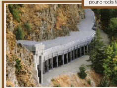
Rockfall hazards in the area west of the west portal of the Mosier Twin Tunnels required construction of mitigation in the form of a 700-foot long rockfall catchment structure.
