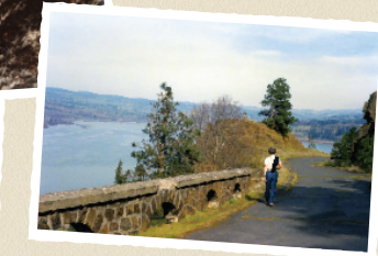
Above and at left: The original highway railings and rubble masonry parapet walls have deteriorated and require restoration. These are photographs of the Rutton Point area prior to the renovations that have been completed in that section of the State Trail.
