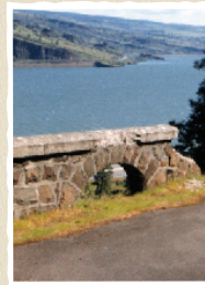
Much of the remaining remnants of the old highway have been utilized as a rock catchment area for I-84
