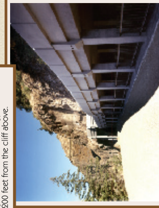
Fascia panels and the colored concrete were included as part of the design of the rock catchment structure to lessen visual impacts.
