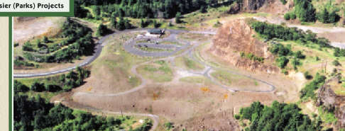
The construction of the Senator Mark O. Hatfield West Trailhead on land near Hood River rehabilitated three gravel pits: Kobberg Quarry (photo-center), Hanel Quarry (edge of photo-left) and the George Quarry (edge of photo right).
