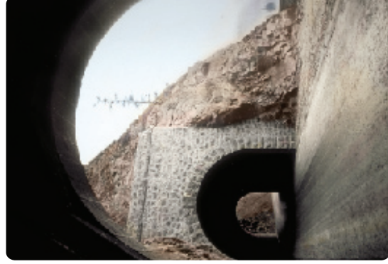
A hand-painted glass slide from ODOT's collection showing the Master Twin Tunnels in the 1930s. The tunnels were widened in 1938 and the rock key ring was replaced with a concrete key ring on both of the mid-tunnel portals.
