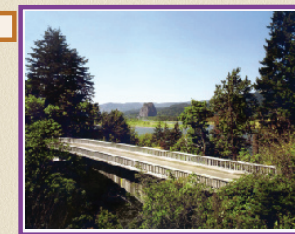
Picture left: Newly constructed rubble masonry parapet rock wall at Bingen Overlook.
