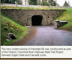
This new undercrossing of Interstate 84 was constructed as part of the Historic Columbia River Highway State Trail Project between Eagle Creek and Cascade Locks.
