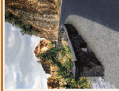
The deteriorated railing on the Toothrock Viaduct was restored to its original condition as part of the project.
