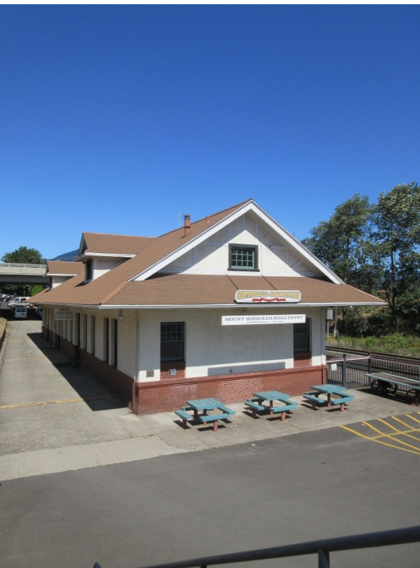
Figure 7.3 O-WR&N Hood River Depot, east elevation, looking northwest
