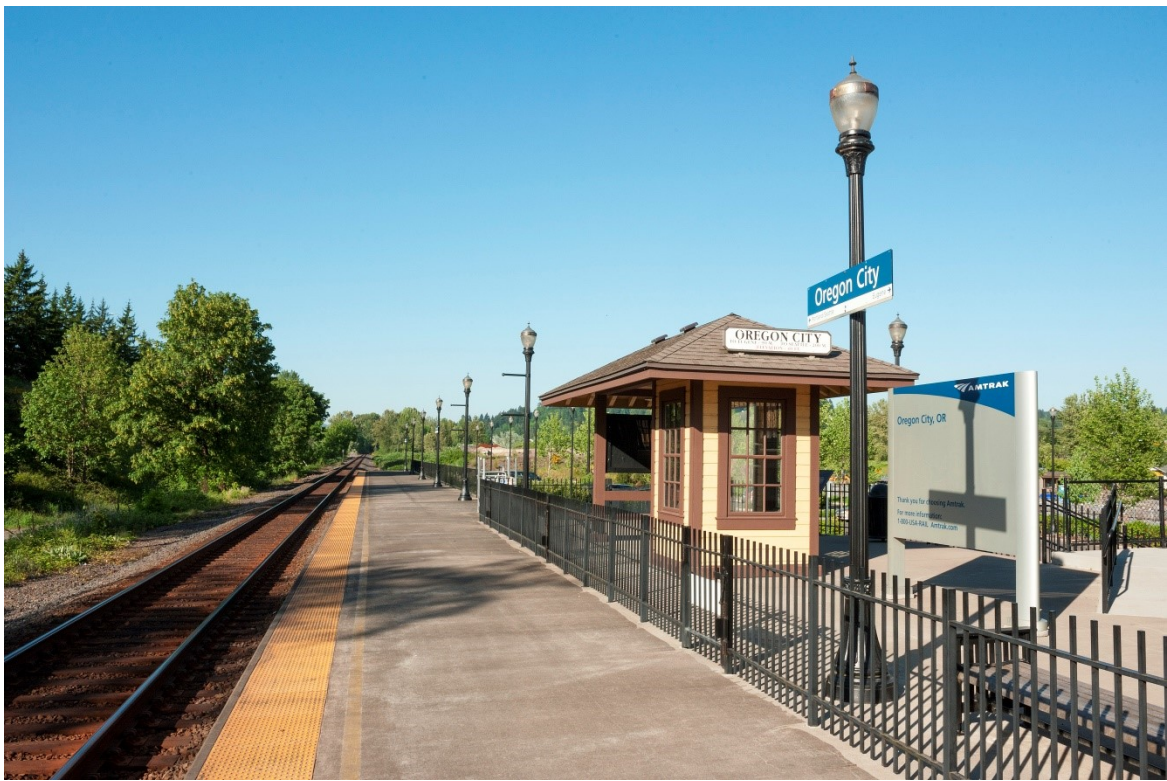
Figure 4.4 The Oregon City station, featuring tactile warning edges, appropriate signage, lighting, and shelter.
