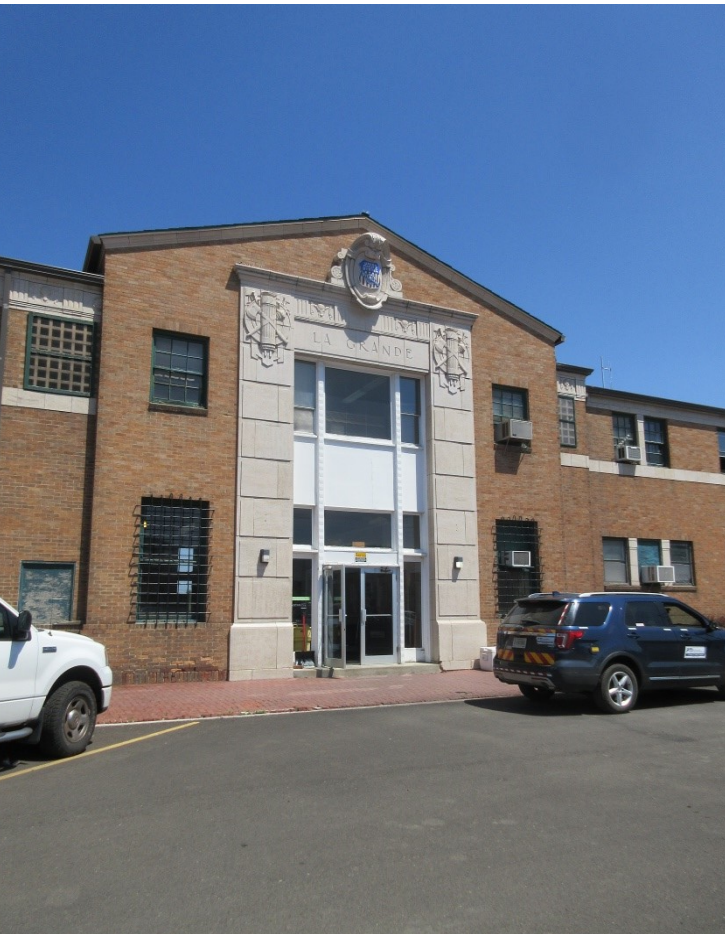
Figure 11.1 La Grande depot, front façade.
