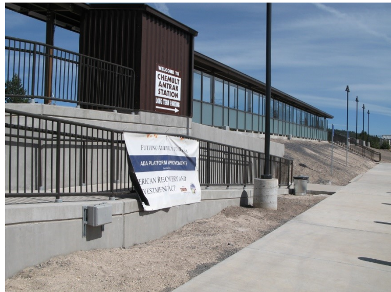
Figure 4.3 New station shelter and ramp at Chemult.
