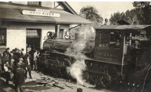
Figure 7.1 Locomotive crashed into the O-WR&N depot in Hood River. (Historic Hood River)
