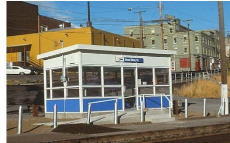
Figure 7.2 Amtrak shelter at Hood River in 1977 (trainweb.org)
