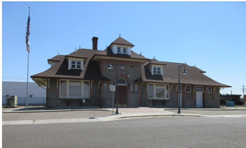
Figure 13.1 OSL depot, front façade, looking east.
