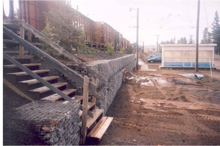
Figure 4.2 Chemult station prior to reconstruction project.
