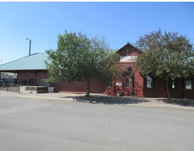
Figure 12.2 SVRy depot, front façade.
