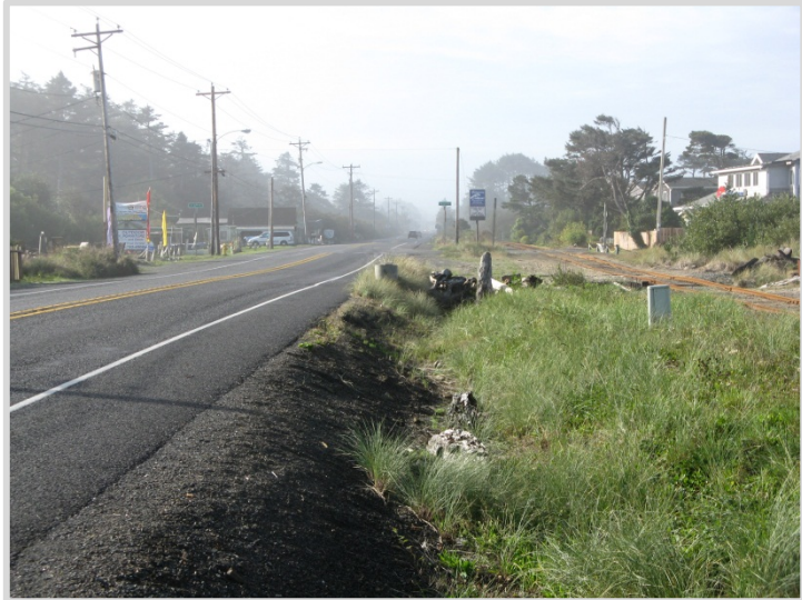
Driftwood remains in the ODOT right-of-way from past storm surge events.
