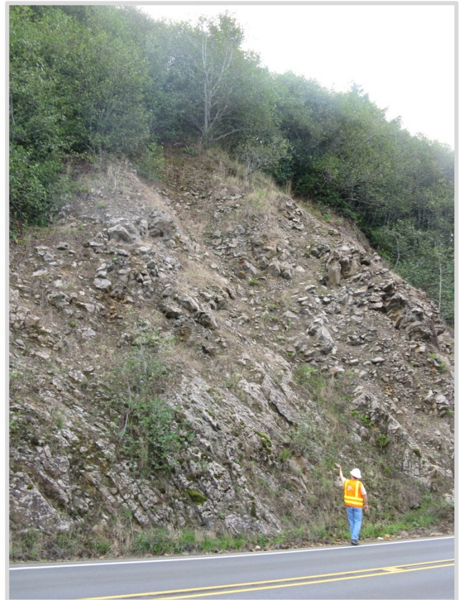
Rock fall site located north of the Jetty Creek landslide complex.
