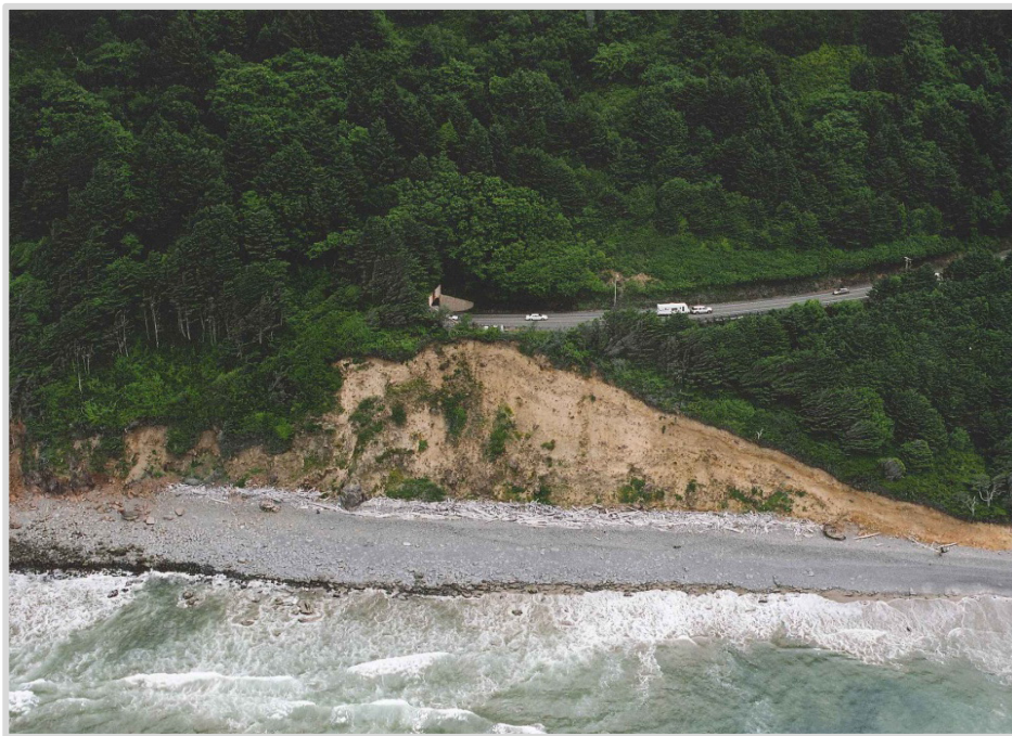
The eroding coastal bluff at Arch Cape tunnel.
