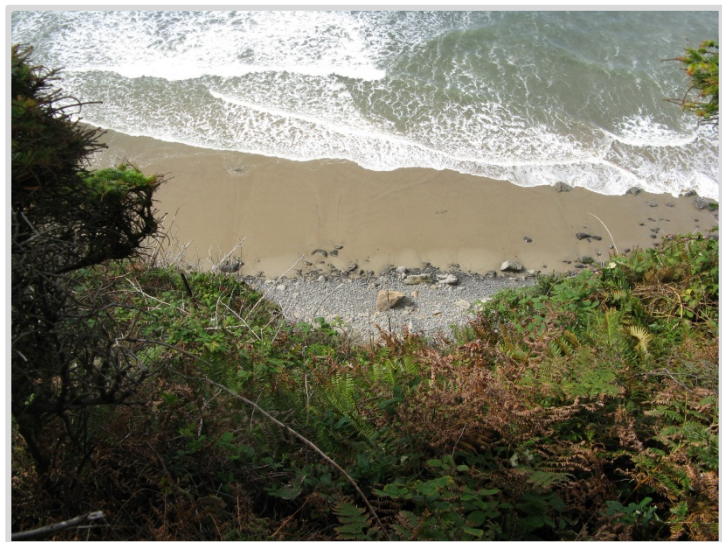
The beach below the steep 100-foot coastal bluff at Arch Cape.
