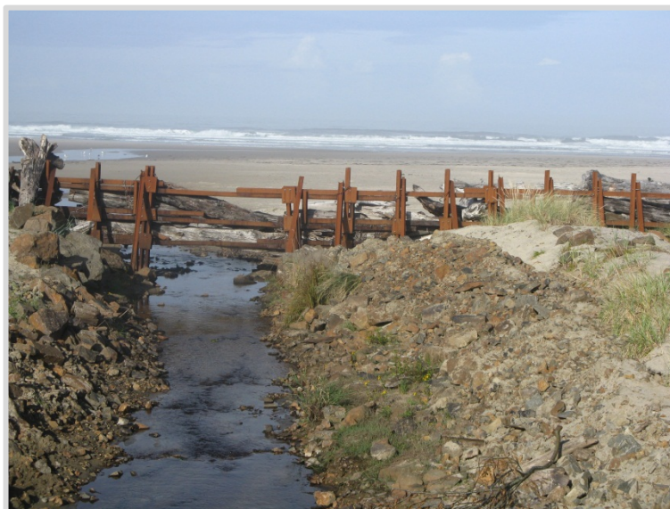
The debris rack at the Salt Air Creek beach outfall.
