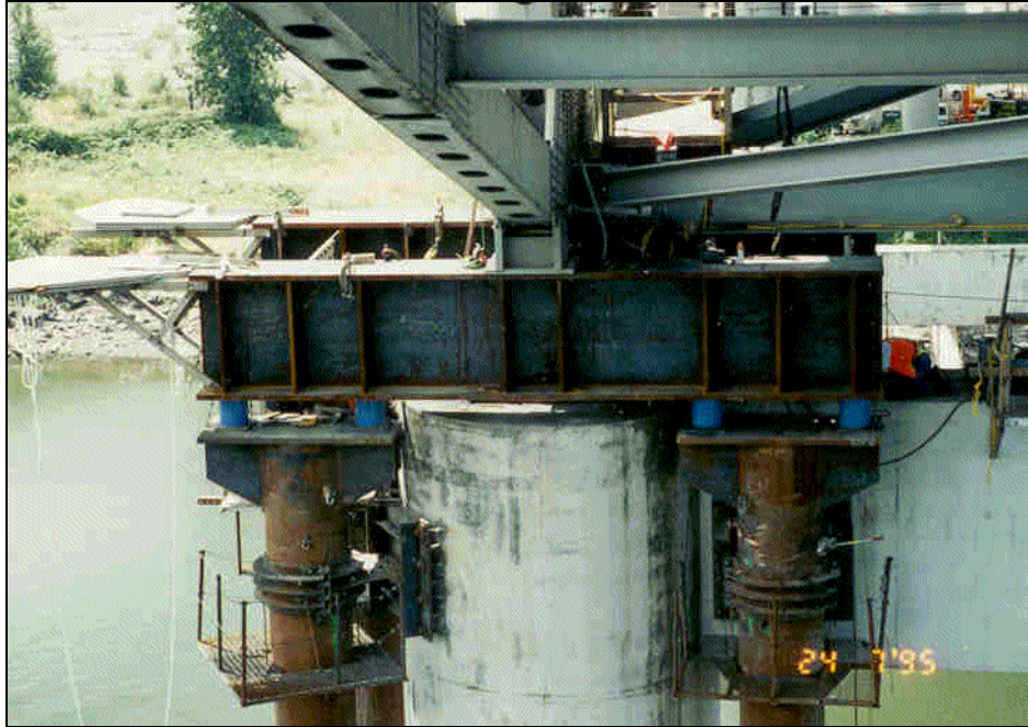
Figure 3.7: The Lifting Assembly for Piers #3 and #4
