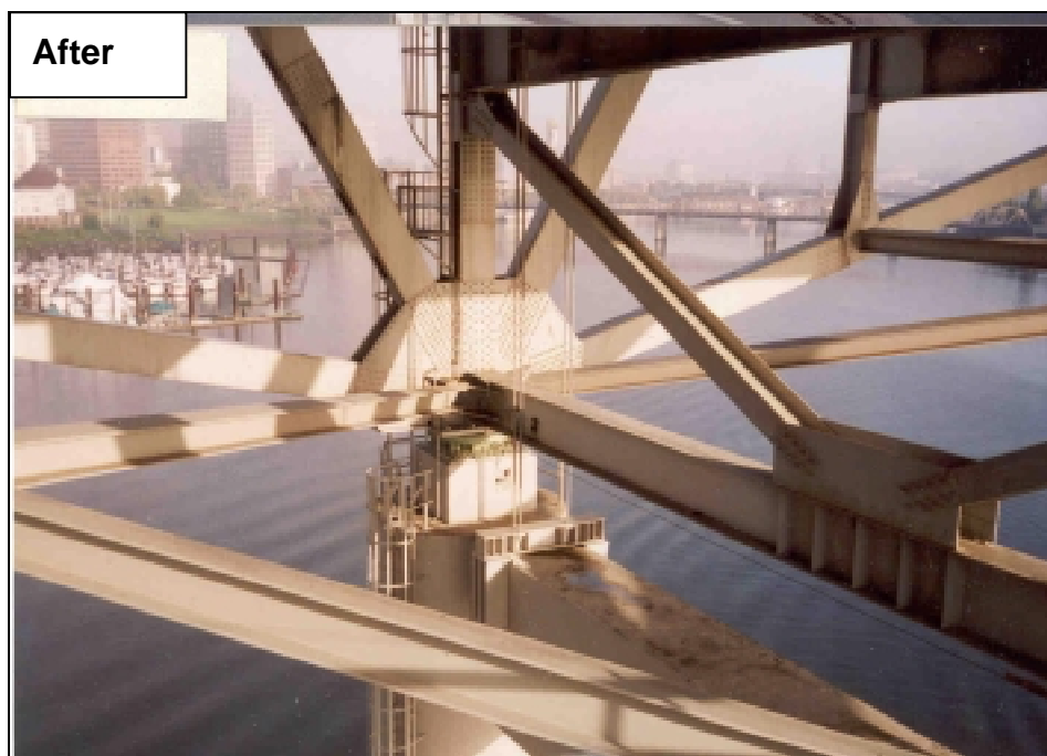
Figure 3.10B: New Bearings on Pier #4
