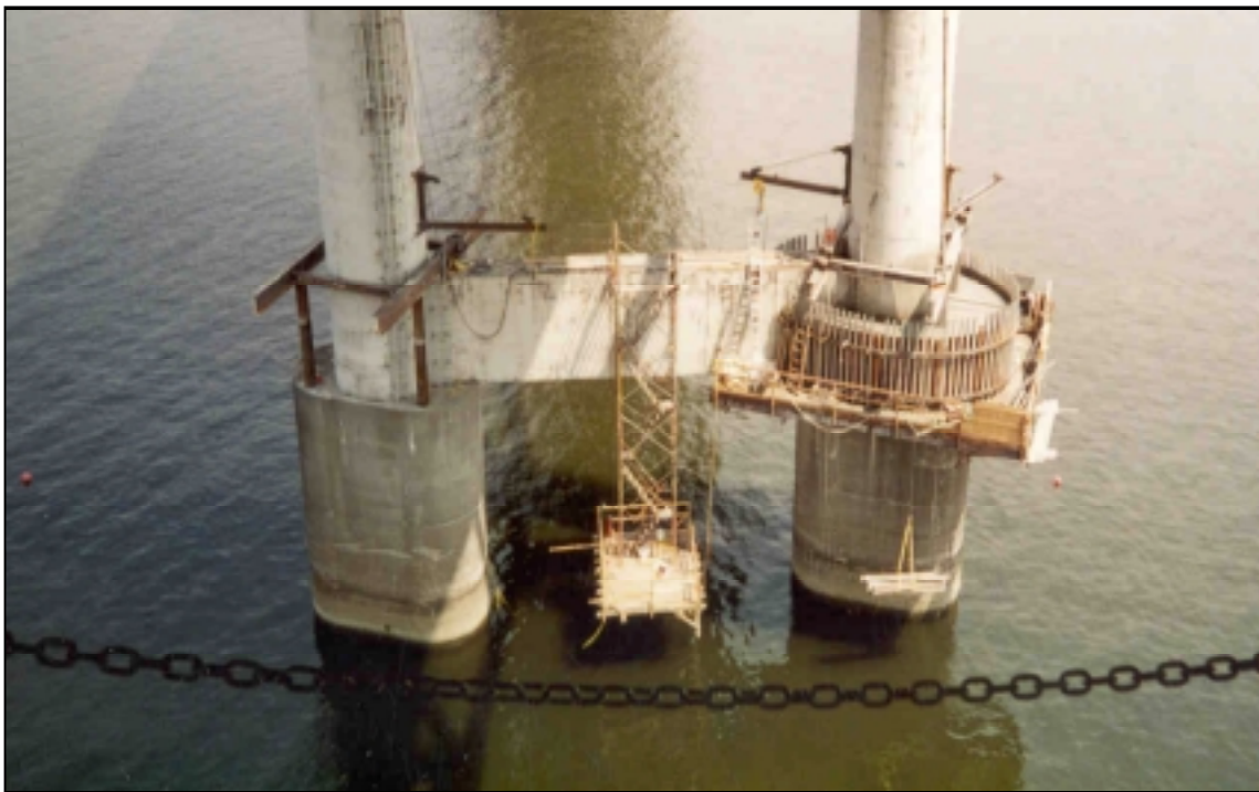
Figure 3.1: Collars Being Constructed Around Pier Columns
