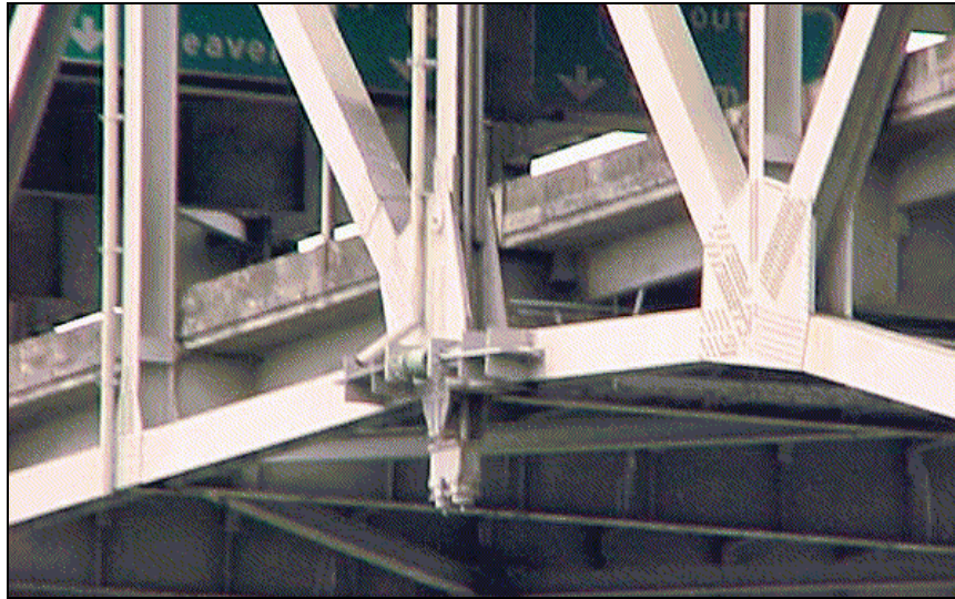
Figure 3.11: Shock Transmission Unit at Panel L13
