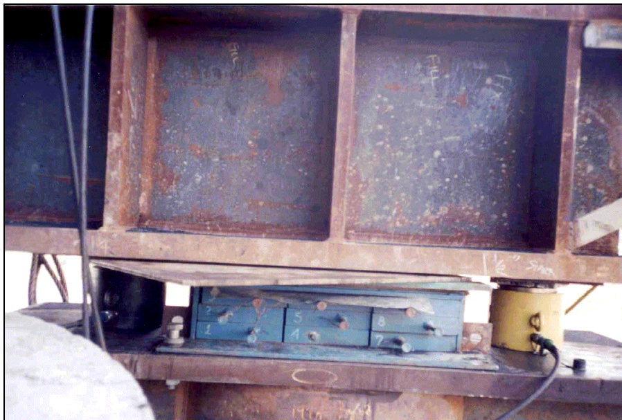
Figure 3.3: The Lifting Assembly for Piers #2 and #5
