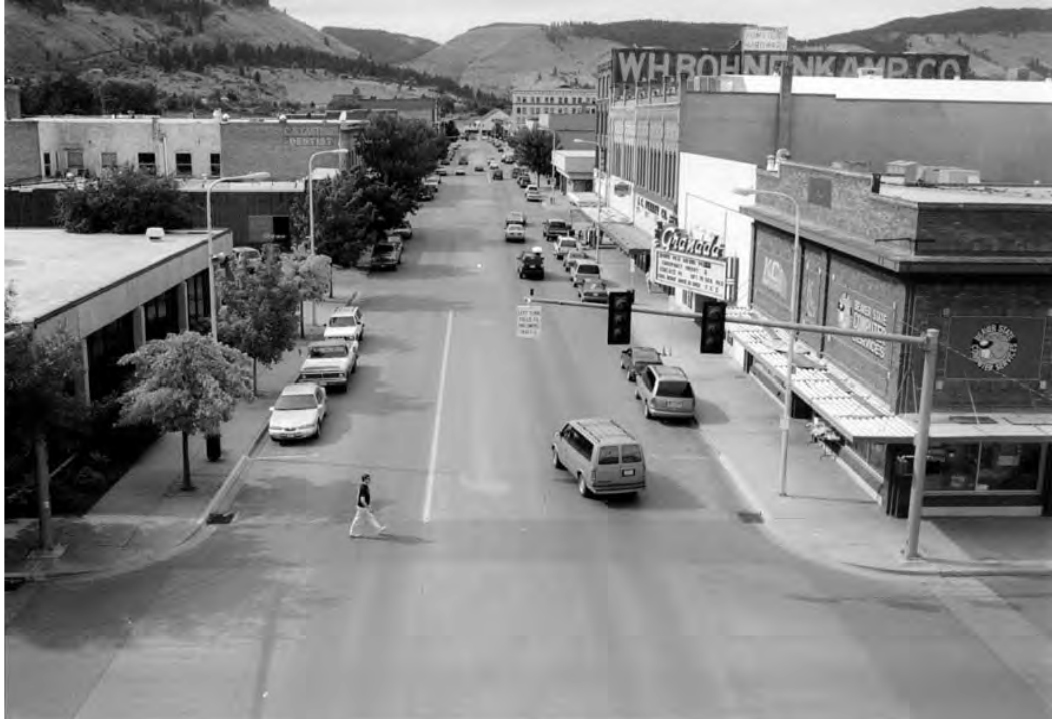
Pedestrian facilities, on-street parking and landscaping are features of Special Transportation Areas like this downtown area on the La Grande-Baker Highway in La Grande
