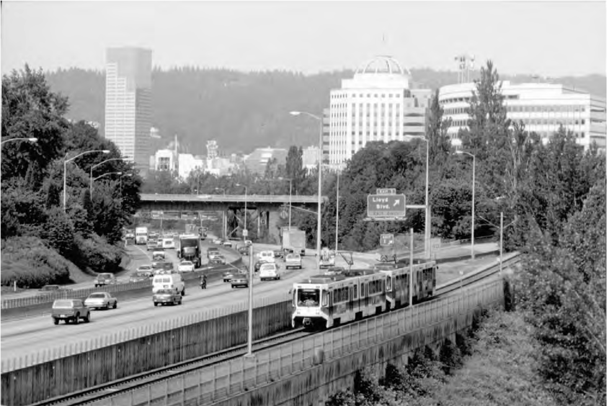
Portland's MAX light rail transit helps relieve congestion in Interstate 84.
