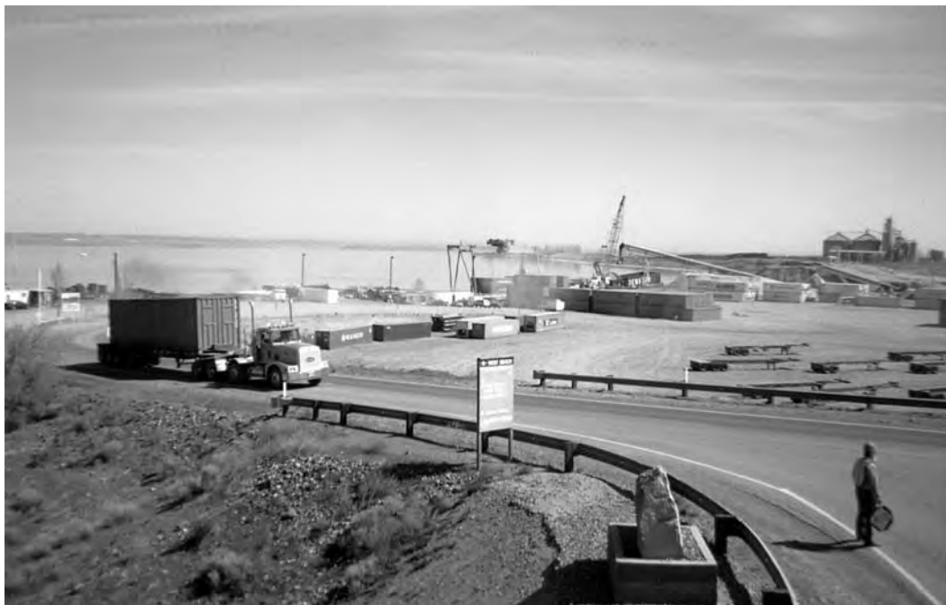
The intermodal connector at the Port of Morrow connects Interstate 84 to port facilities where goods are transferred from truck to barge. (Photo courtesy of Port of Morrow)
