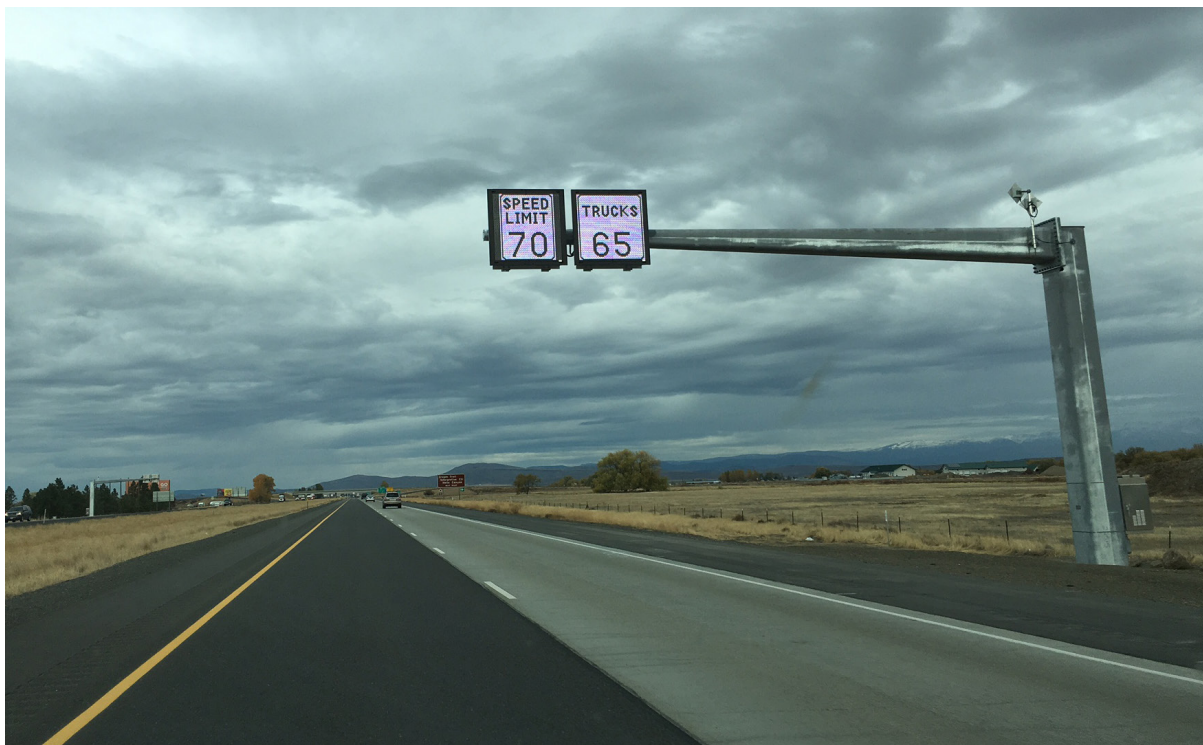
Variable speed limit sign installed along the Baker Valley area
