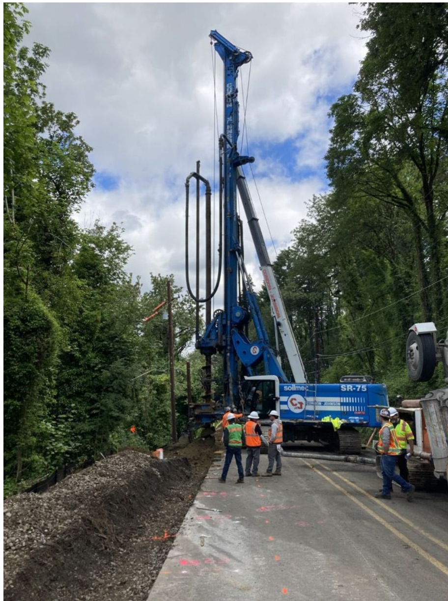
Clackamas County's South End Rd at Milepost 3.8 project. This is an FHWA Emergency Relief funded project. The first picture is drilling the hole for the retaining wall's soldier piles and the second picture is the project completed. - Joel Howie, P.E., Civil Engineering Supervisor, Clackamas County
