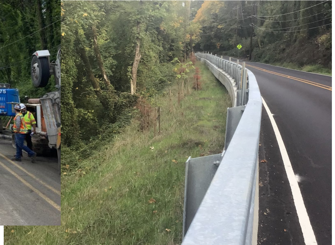
Clackamas County's South End Rd at Milepost 3.8 project. This is an FHWA Emergency Relief funded project. The first picture is drilling the hole for the retaining wall's soldier piles and the second picture is the project completed. - Joel Howie, P.E., Civil Engineering Supervisor, Clackamas County
