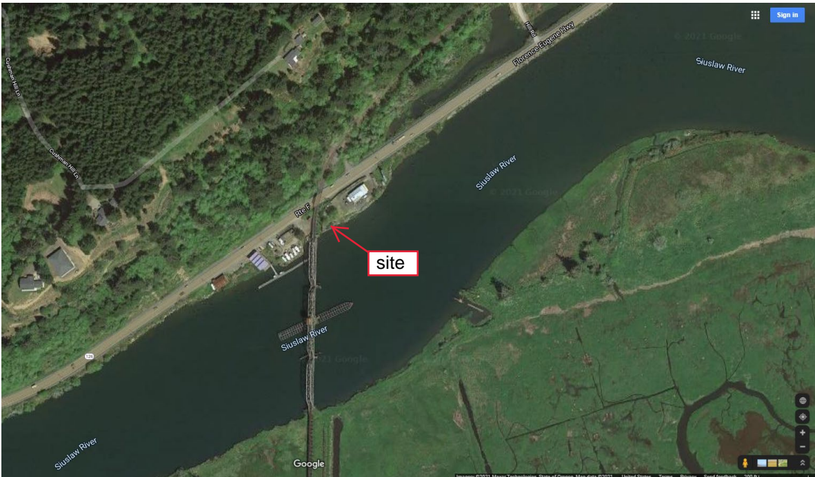
Cushman tide gate Aerial Photograph
