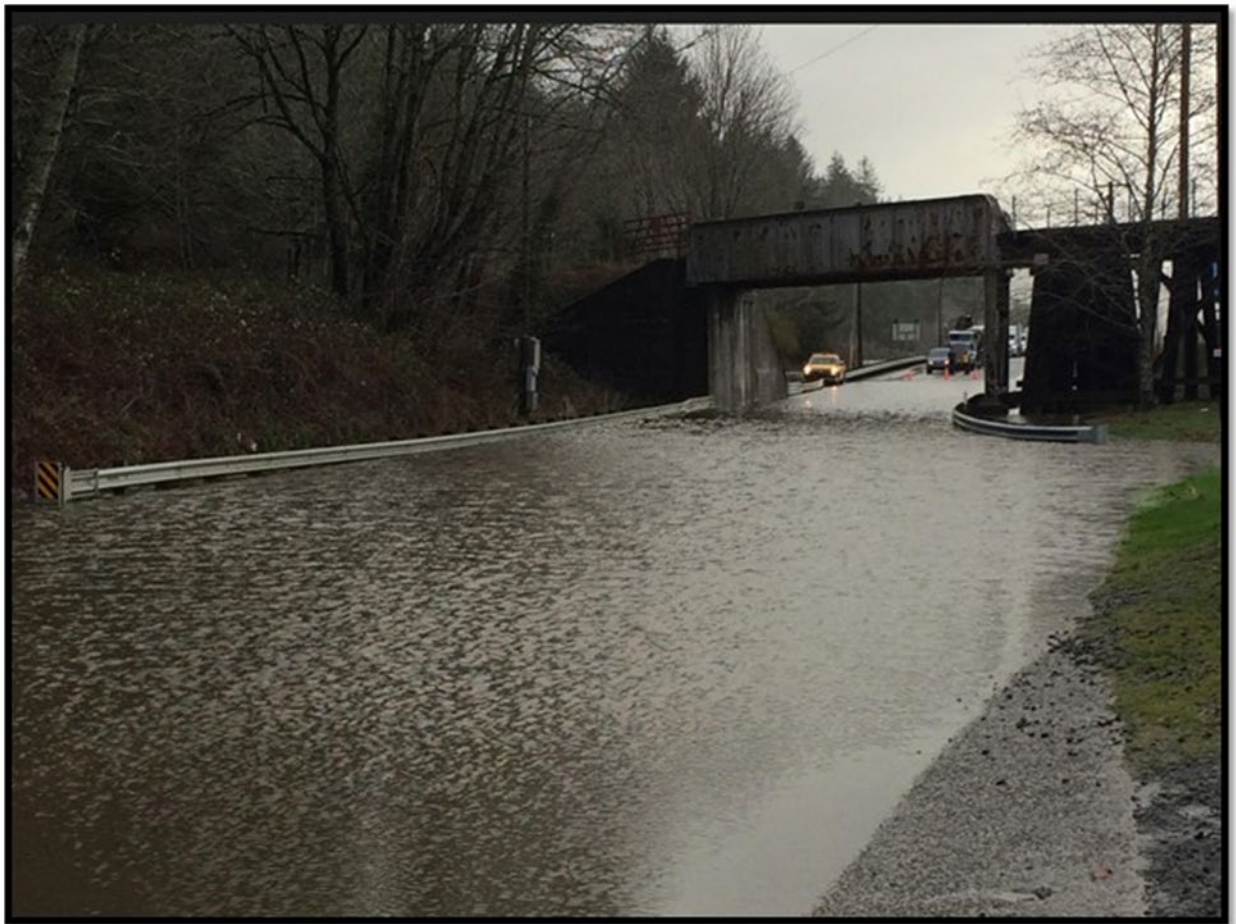
Image 1 – OR 126 (looking east) during flood events.
