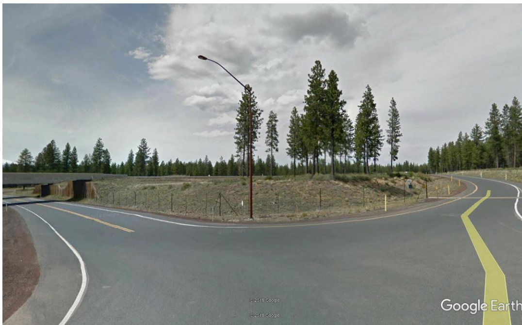
Figure 4.1. South end of exclusion fence as it crosses northbound onramp from South Century Drive and abuts the overpass abutment under U.S. Route 97.
