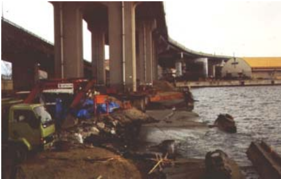
Figure 2.28: Dai-ni Maya Ohashi Bridge
