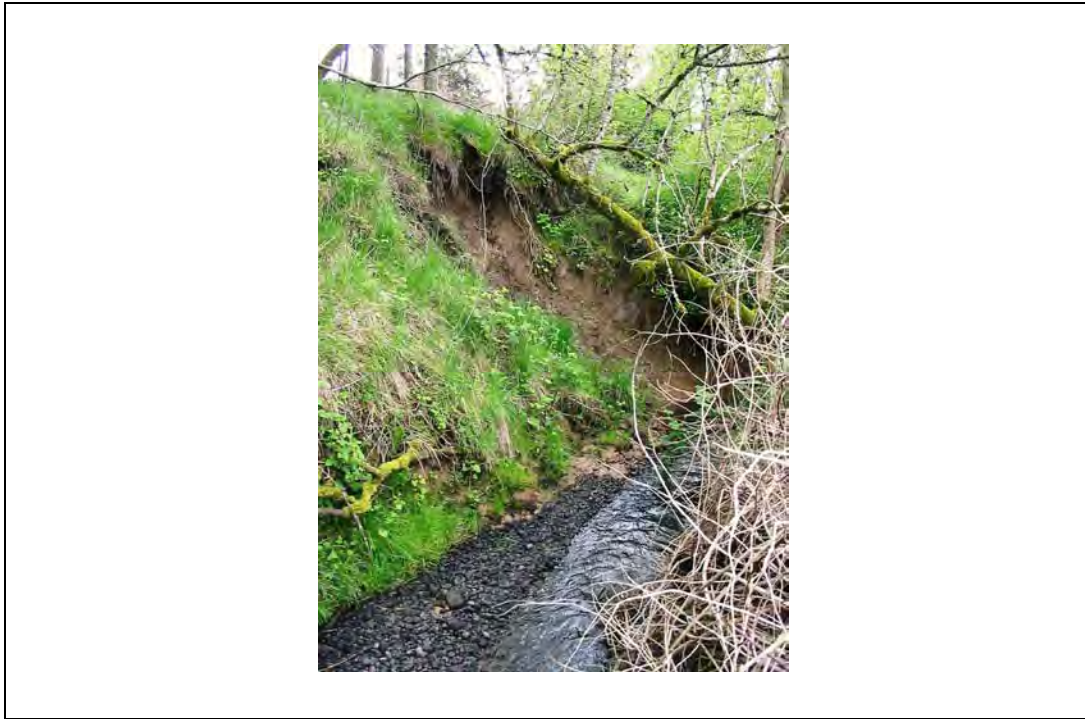
Figure 6-1. Bank erosion on Bronson Creek, Washington County, Oregon. Herrera Environmental Consultants.
