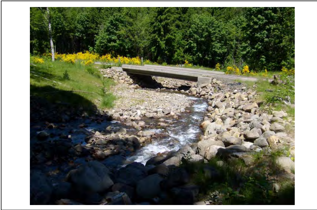
Figure 6-7. Aggradation upstream of a small creek in rural King County, Washington. Herrera Environmental Consultants.
