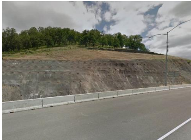
FIGURE 8-6 SHOTCRETE AND SOIL NAIL WALL ON I-5
