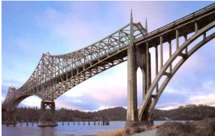
FIGURE 1-3 CONDE McCULLOUGH BRIDGE ON HWY 101 AT COOS BAY
