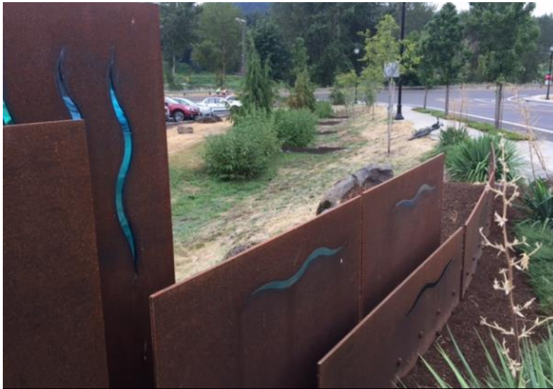
Weathering steel art installation and water quality facility along Hwy 99E in Oregon City
