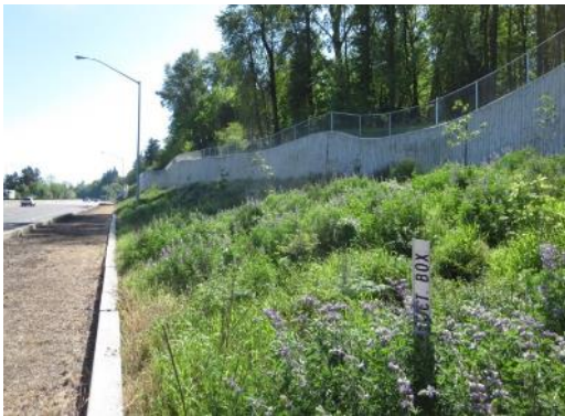
FIGURE 8-17 IOWA ST. RETAINING WALL ON I-5 THROUGH SW PORTLAND
