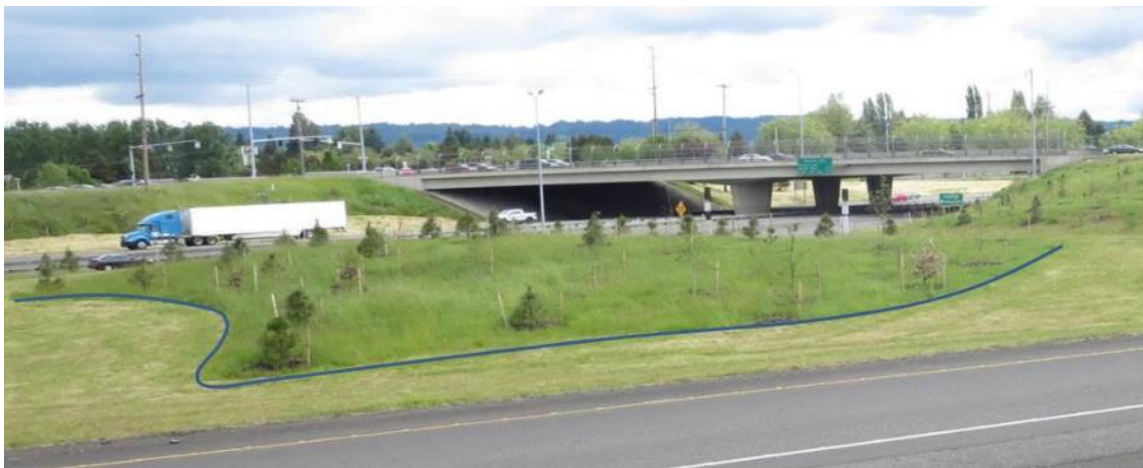
FIGURE 0-5 RUN-OUT AND RECOVERY ZONE
