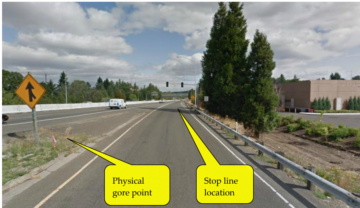
Figure 13-3 | Physical Constraints (Barrier on Left Side) - Requires Overhead Mount
