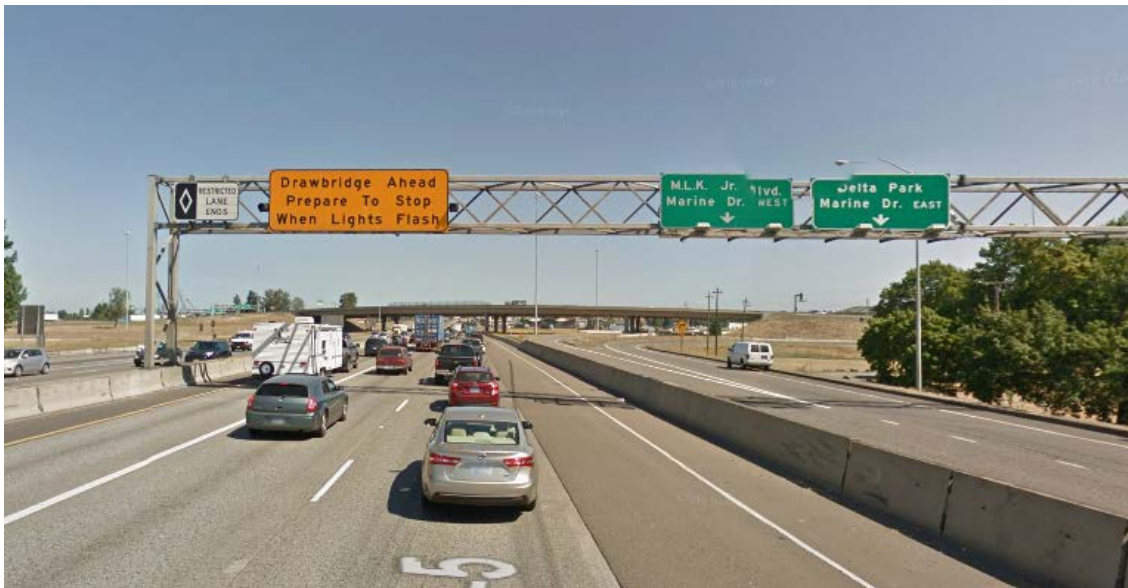
Figure 23-15 | Columbia River NB: 1 st Warning Device
