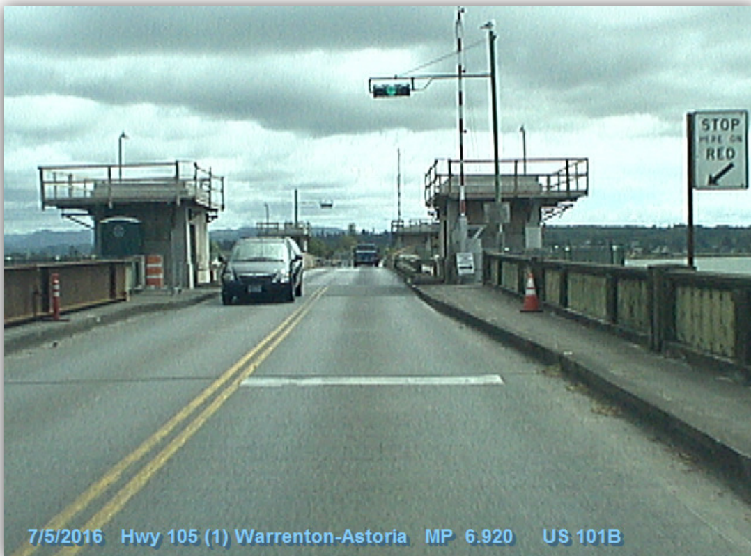
Figure 23-1 | Non-Compliant Existing TCD: Single Signal Head to Stop Traffic Mounted Horizontally
