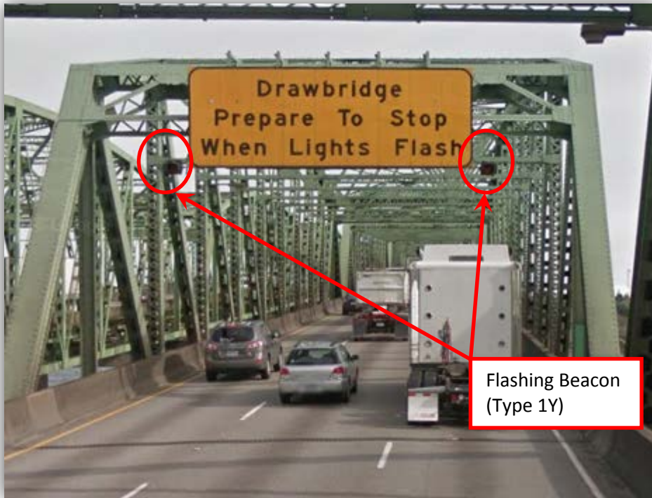
Figure 23-16 | Columbia River NB: 2 st Warning Device
