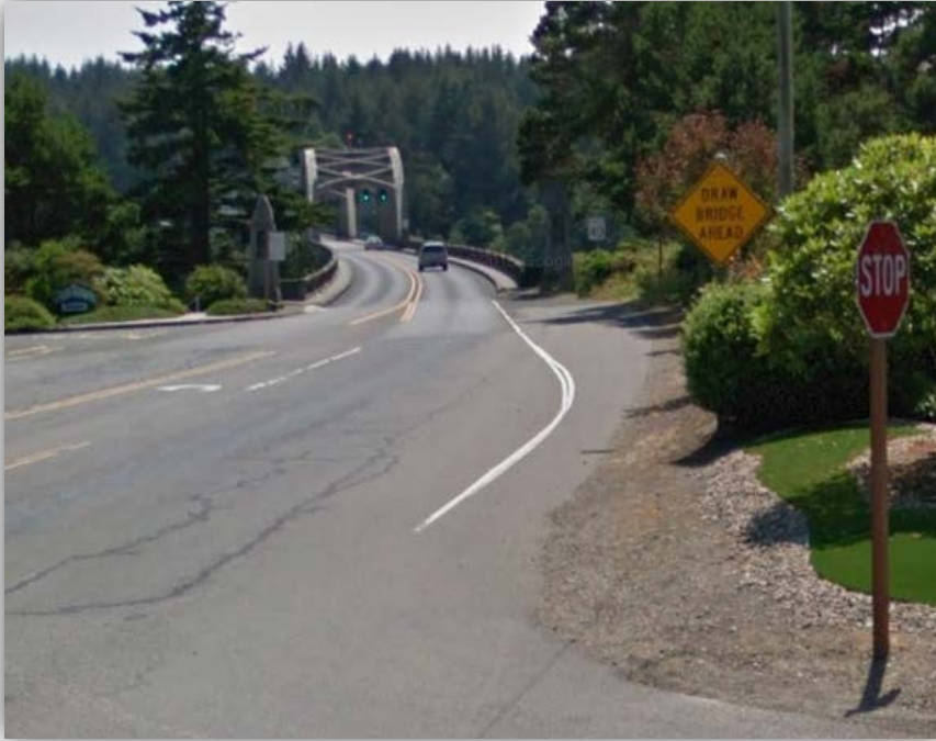
Figure 23-6 | Non-Compliant Existing TCD: Outdated Signs, Example 1
