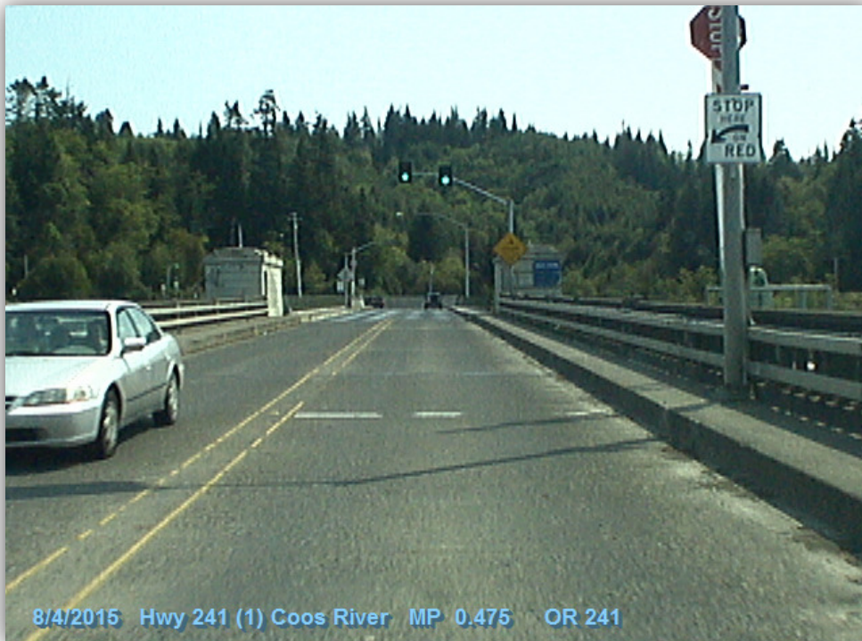
Figure 23-3 | Non-Compliant Existing TCD: Mounting a STOP sign to the warning gate
