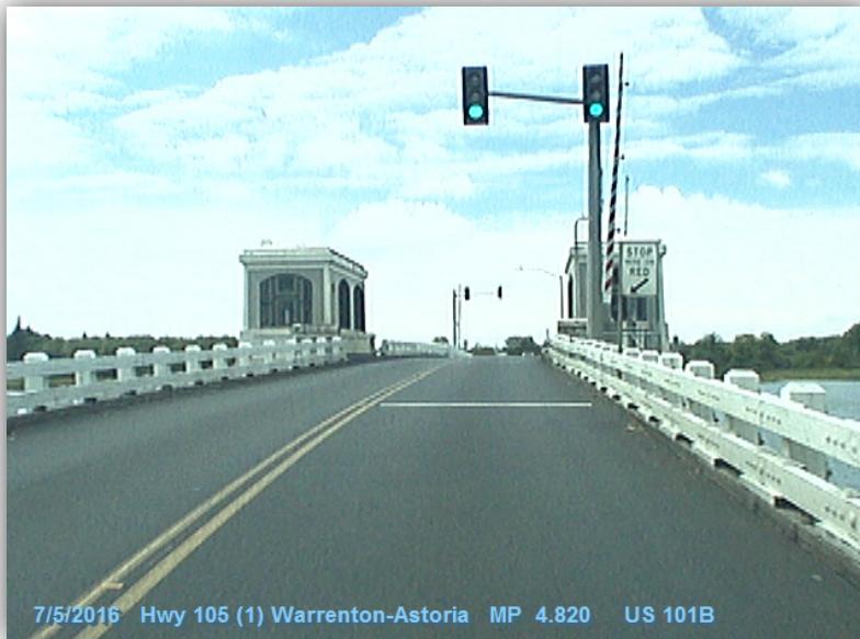
Figure 23-11 | Signal Heads and Sign Custom Mounted on Bridge Structure
