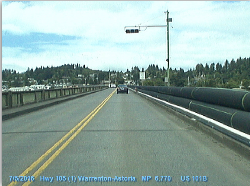
Figure 23-5 | Non-Compliant Existing TCD: Single Advance Signal Head, Example 2
