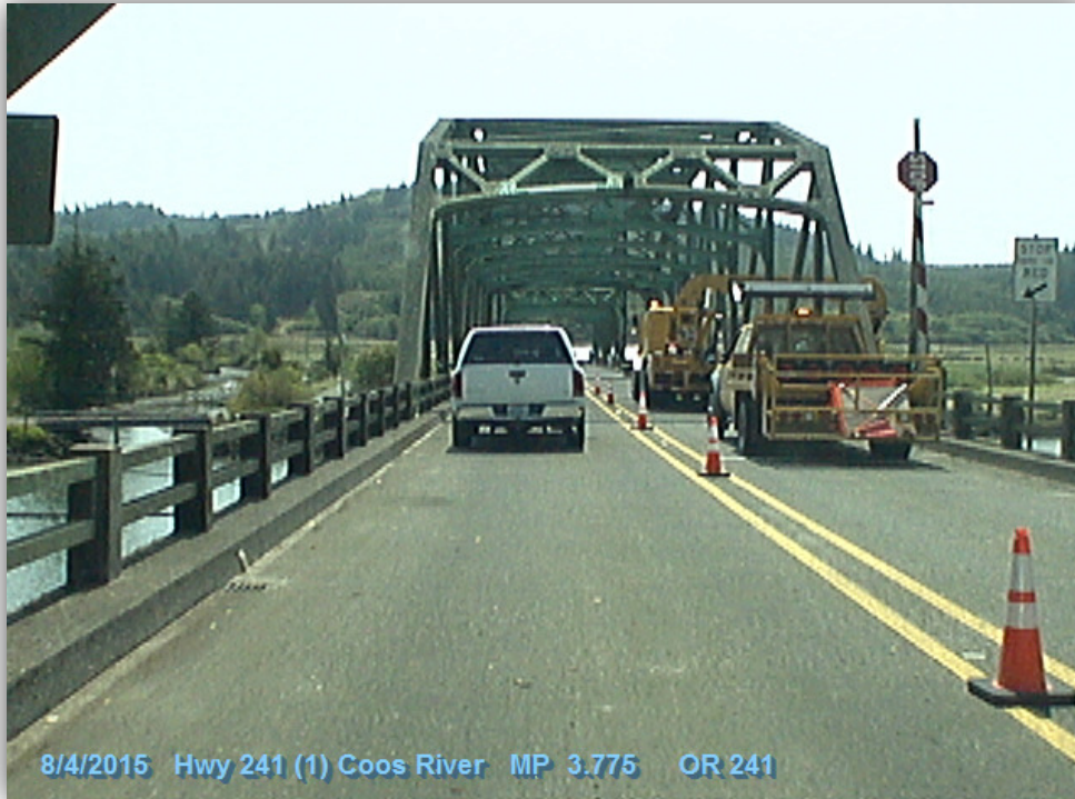
Figure 23-2 | Non-Compliant Existing TCD: Use of Only Bridge Warning Gates with No Traffic Signals
