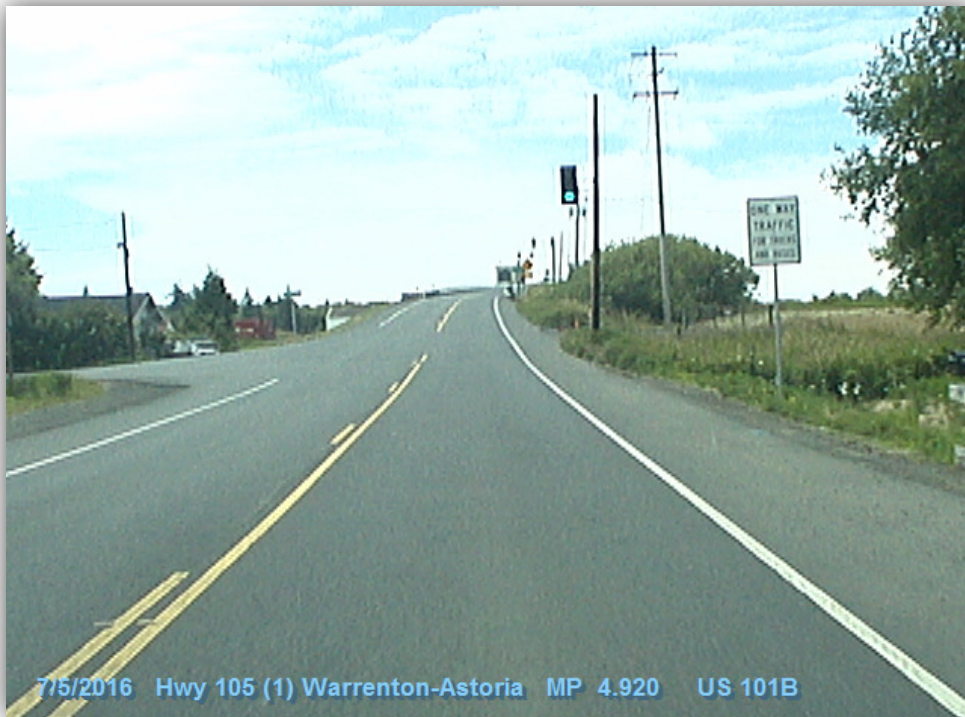
Figure 23-5 | Non-Compliant Existing TCD: Single Advance Signal Head, Example 2
