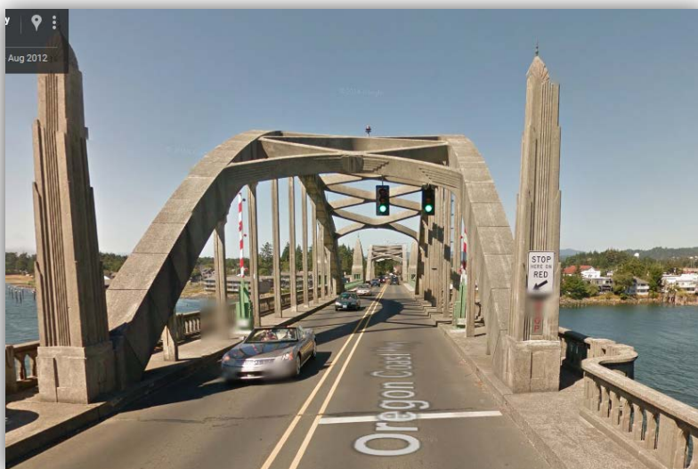
Figure 23-11 | Signal Heads and Sign Custom Mounted on Bridge Structure
