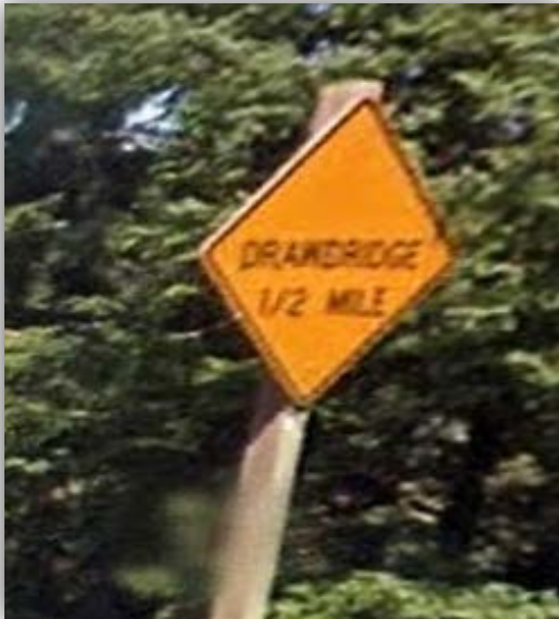
Figure 23-7 | Non-Compliant Existing TCD: Outdated Signs, Example 2
