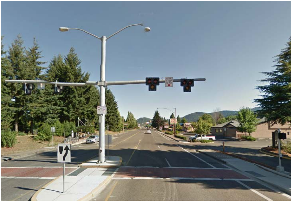
Figure 12-20 | Pedestrian Hybrid Beacon – Overhead Mounted, Example 1
