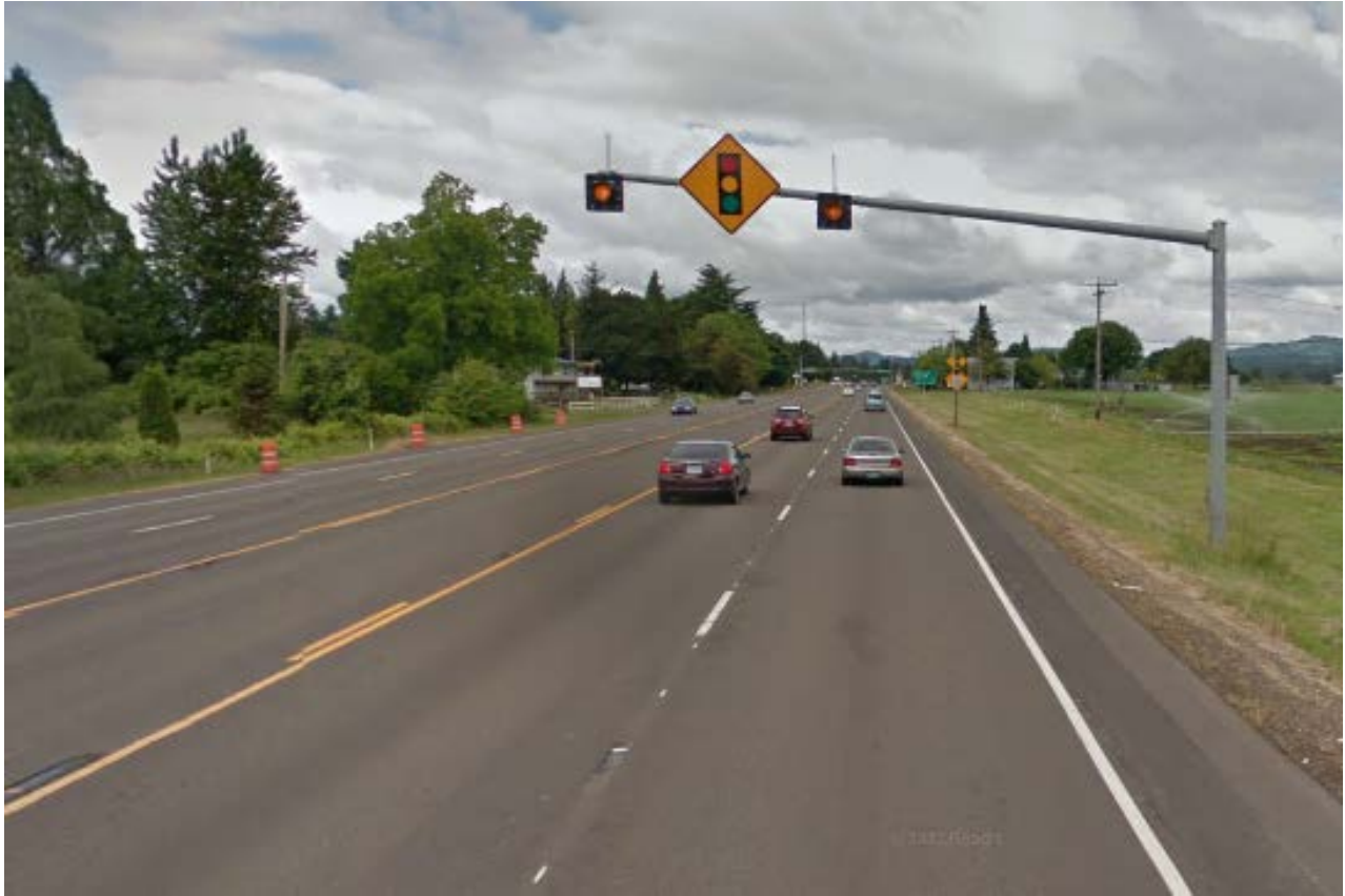
Figure 12-4 | Warning Beacon for a Warning Sign, Overhead
