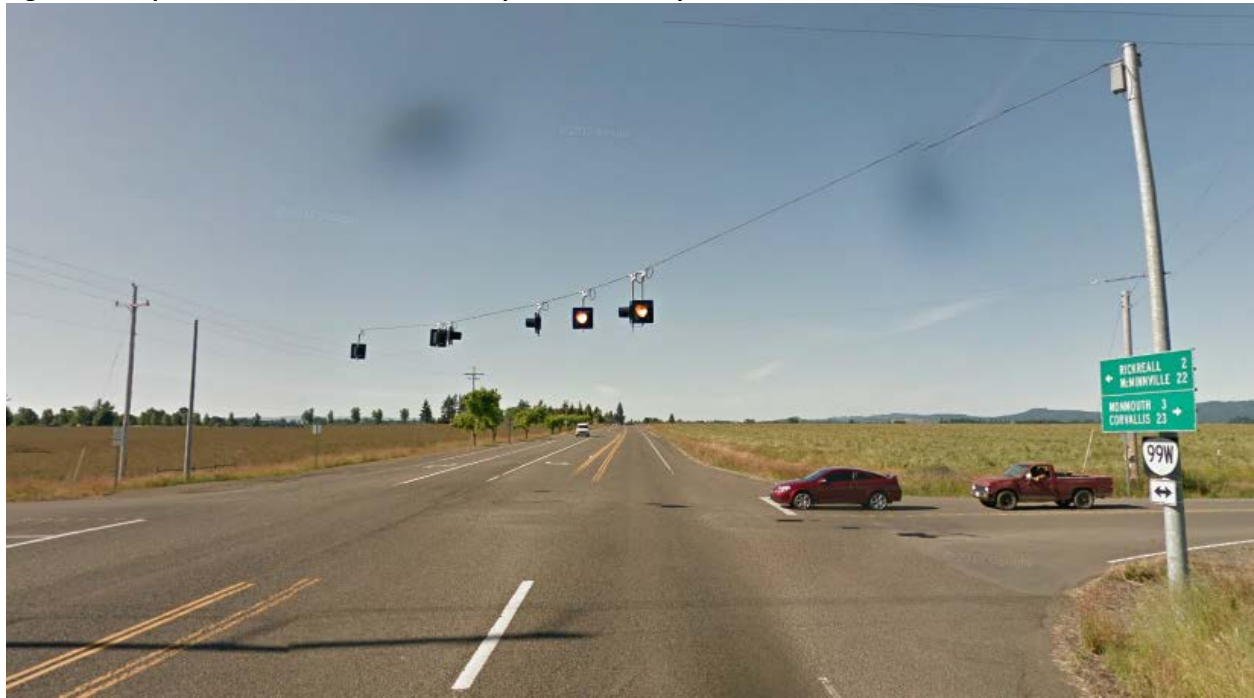
Figure 12-17 | Intersection Control Beacon, Span Wire, Example 3
