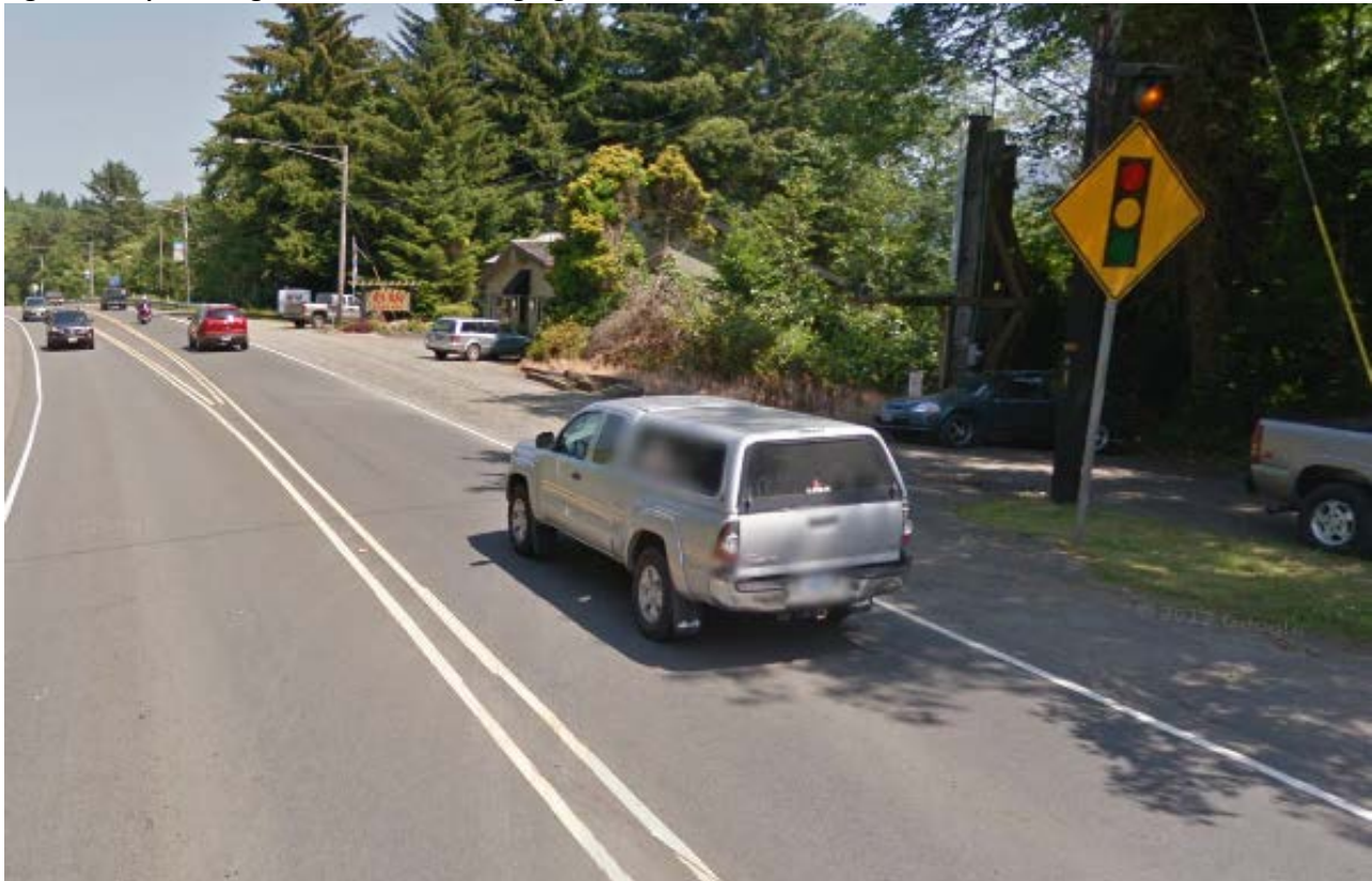
Figure 12-3 | Warning Beacon for a Warning Sign, Post Mounted
