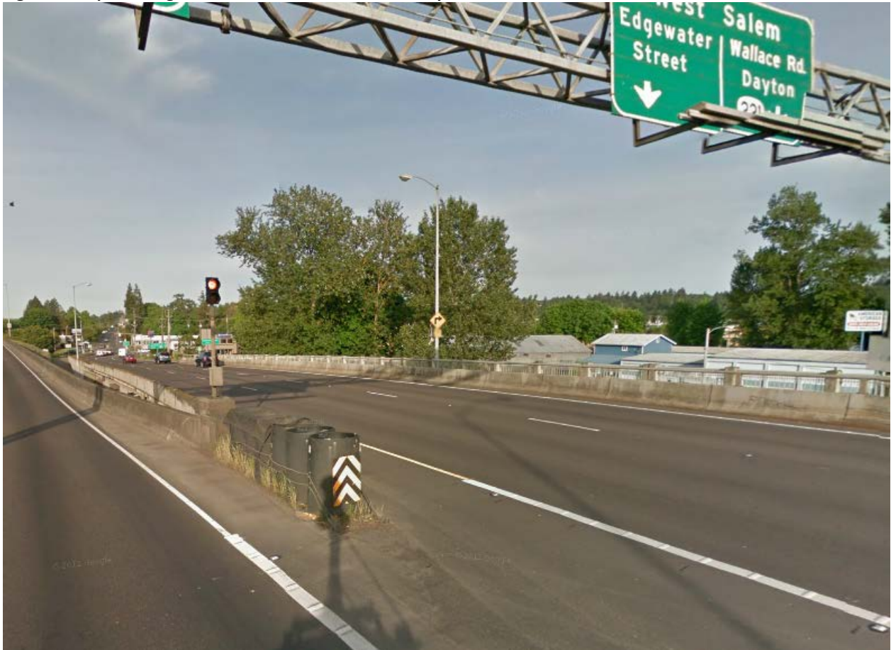
Figure 12-1 | Warning Beacon for an Obstruction, Example 1
