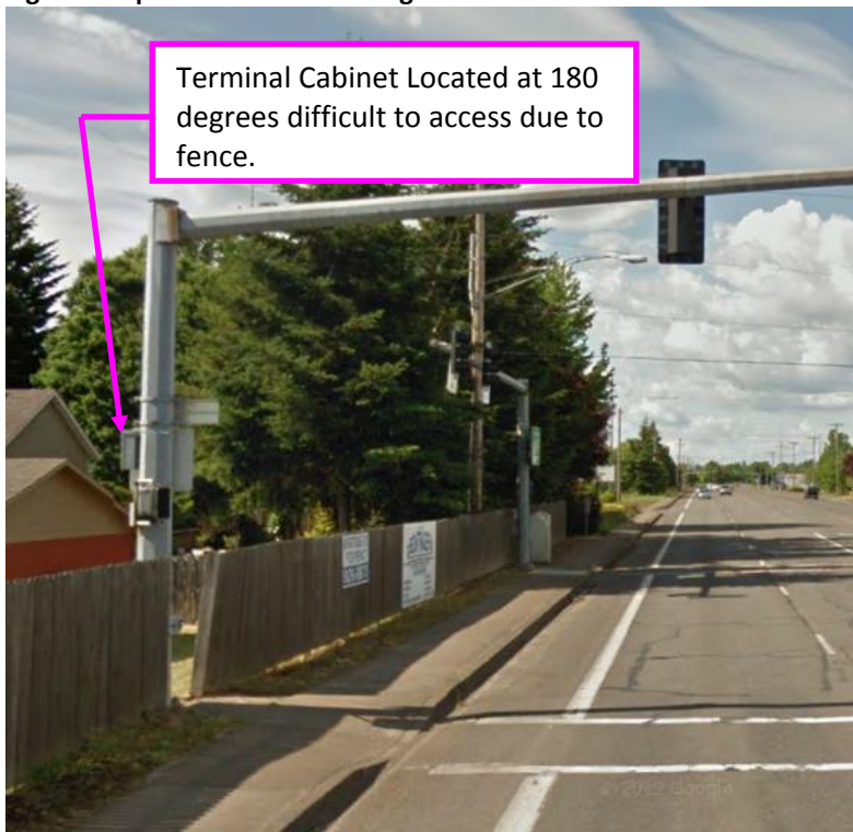
Figure 9-8 | Terminal Cabinet Degrees: Access Obstruction
