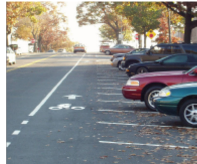
Back-in Diagonal Parking Improved Visibility to Oncoming Vehicles and Bicyclists
