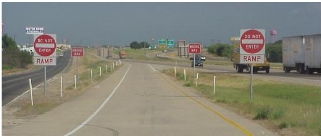
Figure 3-6: Supplemental One Way (Top) And Ramp (Bottom) Signs To Do Not Enter Signs, (Cooner Et Al. 2003).
