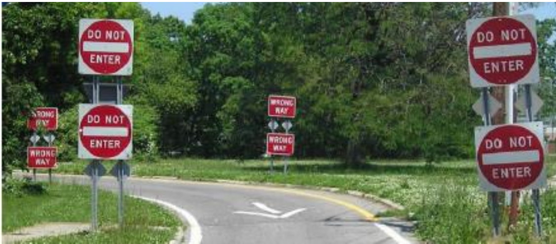
Figure 3-2: Larger Signs and Additional Signs to Deter Wrong-Way Drivers, (NTSB 2012).
