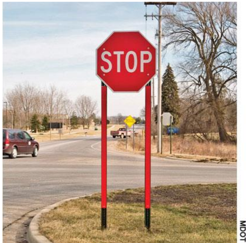
Figure 5-4 Red Reflective Material on STOP Sign Post
