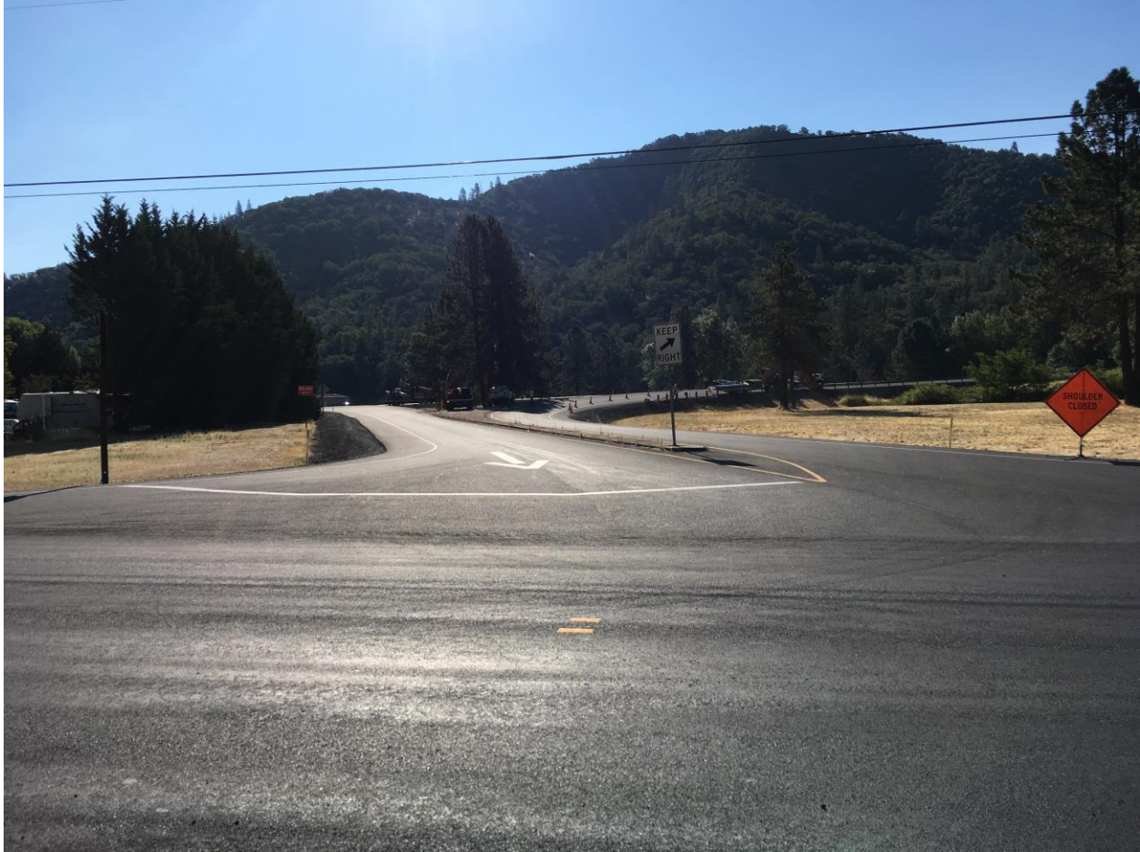
Figure 5-10 Keep Right Sign in Raised Median Separating the Entry and Exit Ramps
