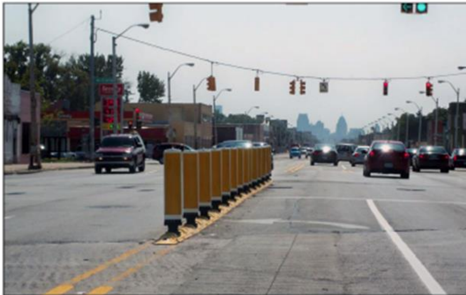
Figure 3-32: Longitudinal Channelizing Devices Prevent Wrong-Way Left-Turn Movement, (Morena and Ault 2013)
