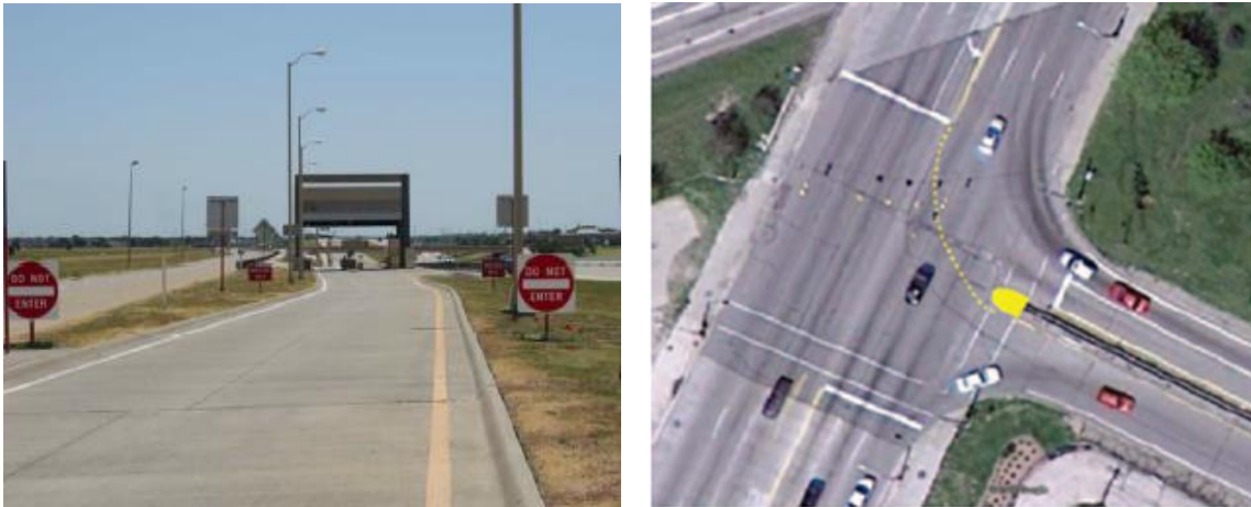
Figure 3-12: Solid Yellow Line on the Left Edge of an Exit Ramp (Left). Dotted Lane Extension, Painted Island in Ramp Intersection, and Stop Line Downstream of Exit-Ramp (Right), (Zhou and Pour Rouholamin 2014a)
