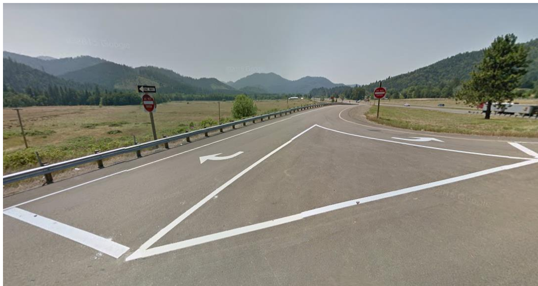
Figure 5-8: Lane Use Arrows on an Exit Ramp
