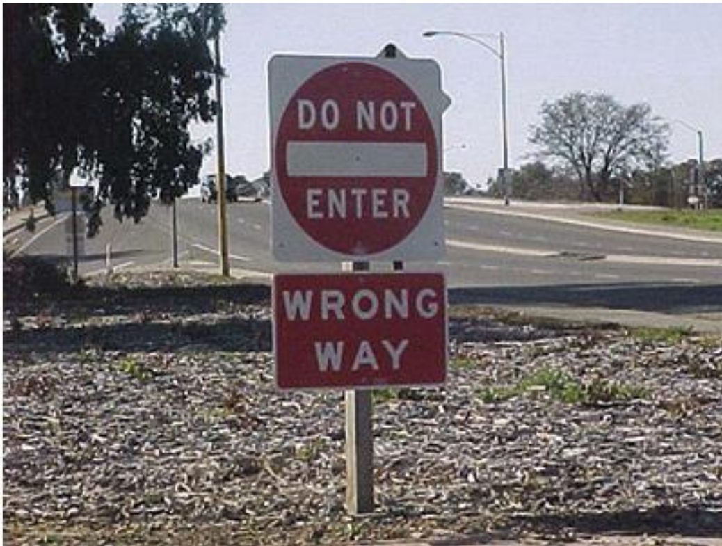
Figure 5-2: Low Mounted DO NOT ENTER (DNE) and WRONG WAY (WW) Signs Used by CalTrans (FHWA)
