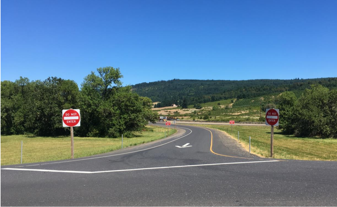
Figure 5-1: DO NOT ENTER (DNE) Sign Pair at Exit Ramp Terminal
