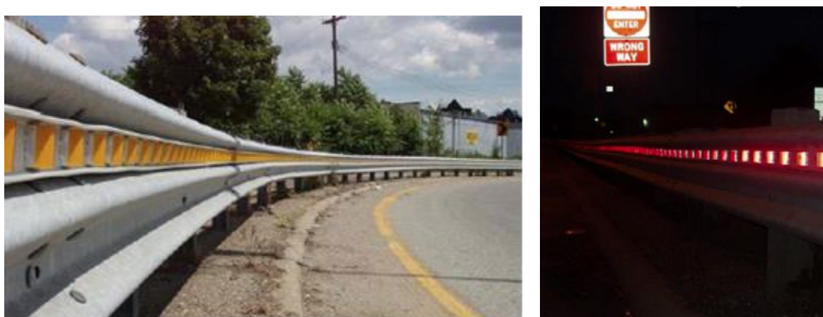
Figure 3-13: Yellow Delineations in Right-Way of Travel (Left Image) and Red Delineations in Wrong-Way of Travel (Right Image) along Exit Ramp Barriers, (Zhou and Pour Rouholamin 2014a)
