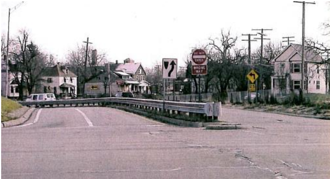
Figure 3-37: Median Barrier Blocks Conspicuity of the Entrance Ramp, (Morena and Leix 2012)
