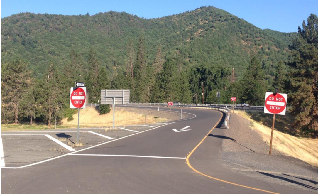
Figure 5-7: Wrong Way Arrow Placed Near DNE Signs at an Exit Ramp
