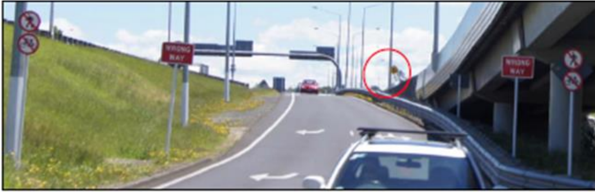
Figure 3-1: Warning Sign for Busway Visible From Off Ramp, (Baisyet et al. 2015)
