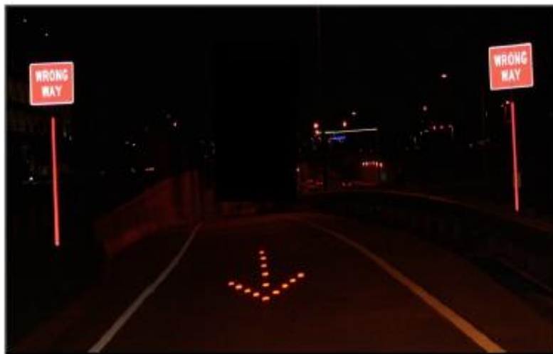
Figure 3-10: Wrong-Way Arrows near Supplemented by RPMs and WW Signs, (Zhou and Pour Rouholamin 2014a)
