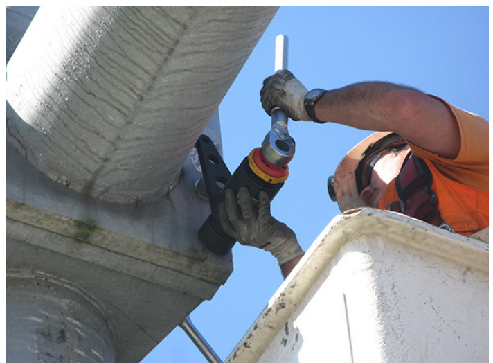
Bolt Tightening with Multiplier (Best practice for achieving proper tensioning)
