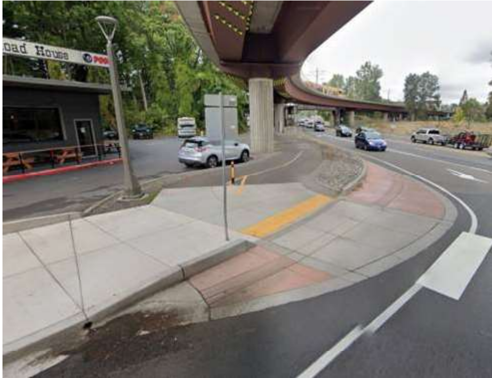
Truck Apron at a Shared Use Path Curb Ramp
