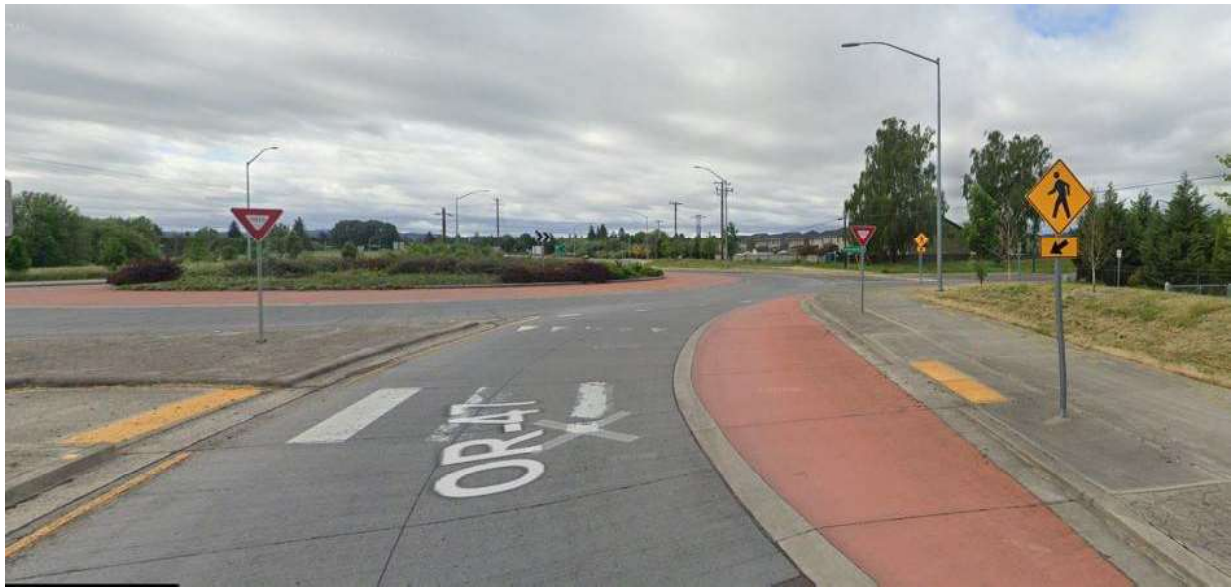
Truck Apron at a Roundabout
