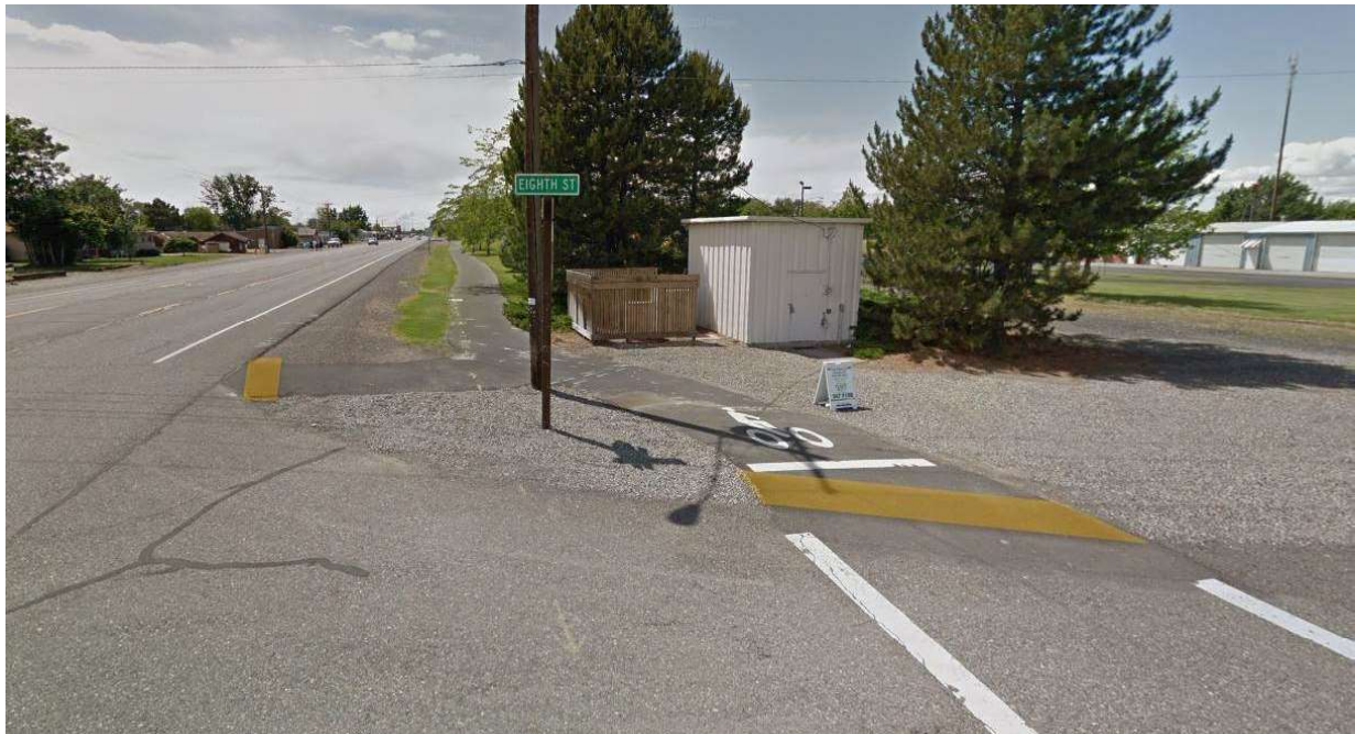
Image of a Curbless Construction for An Asphalt Walkway and Shared Use Path.
