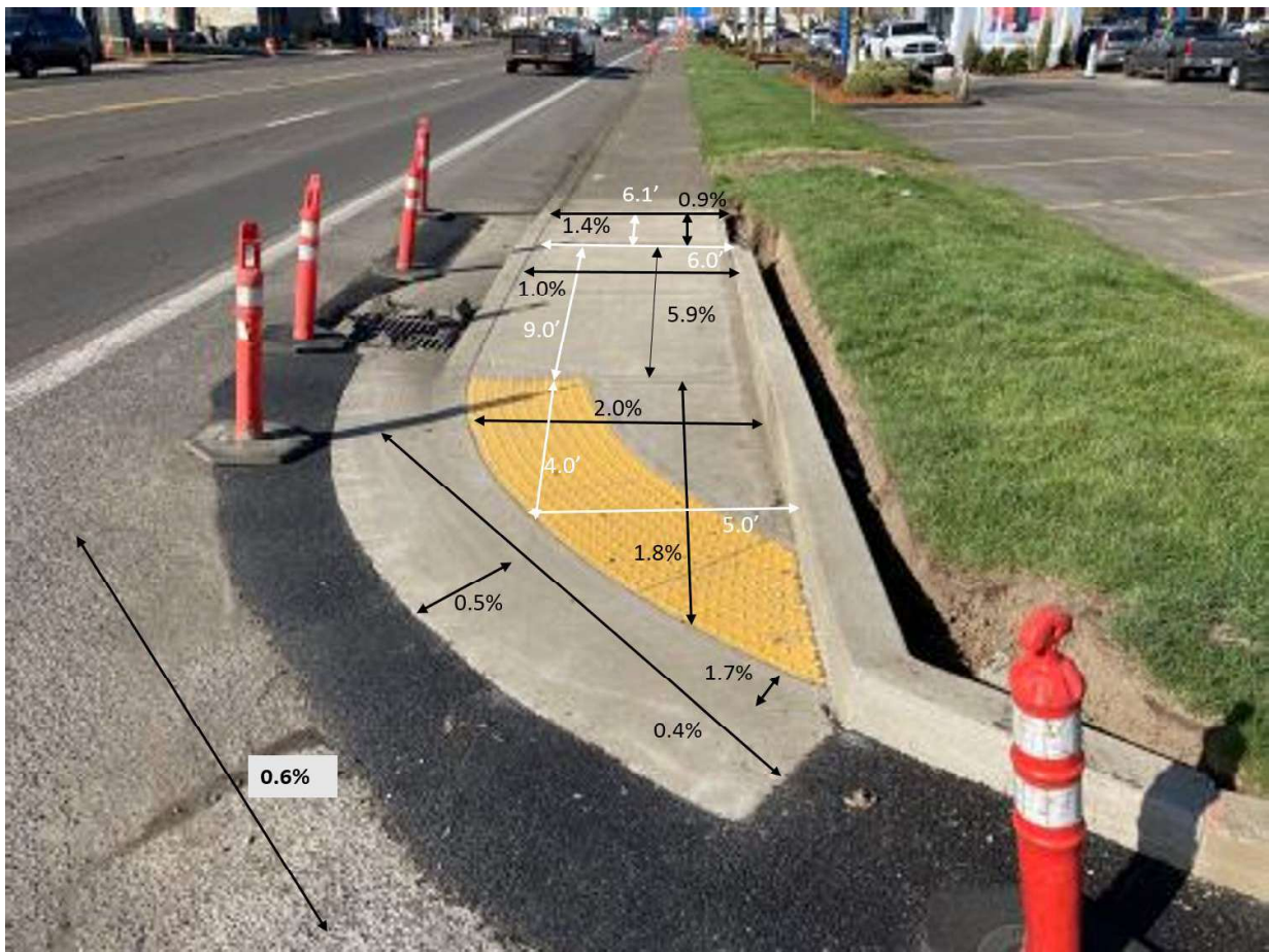
Example 7: Fully Lowered Unique Design Curb Ramp
