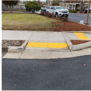
Good Example Photo of Curb Ramp for Inspection Form
