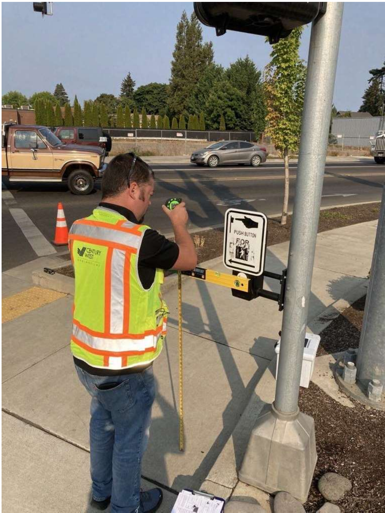
Measuring Push Button Height in the Field
