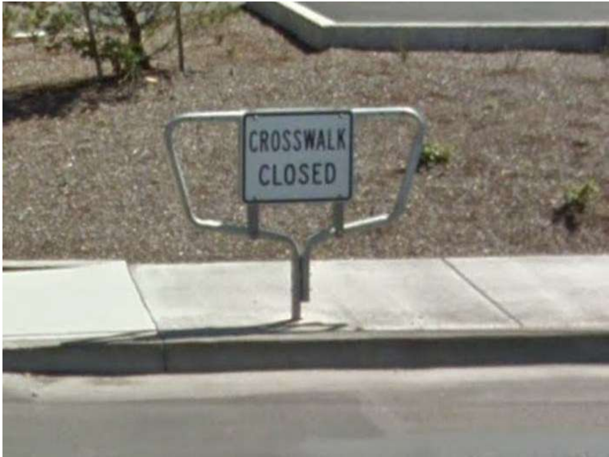
Proper installation of a Crosswalk Closure Support
