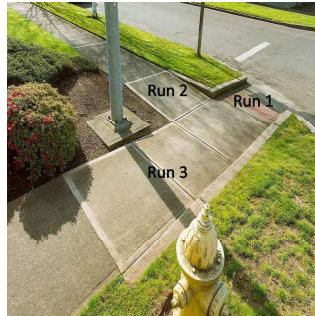
Combination Curb Ramp Numbering Scheme
