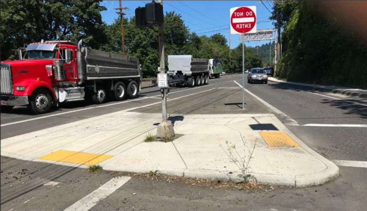
Island with Perpendicular Curb Ramp Systems
