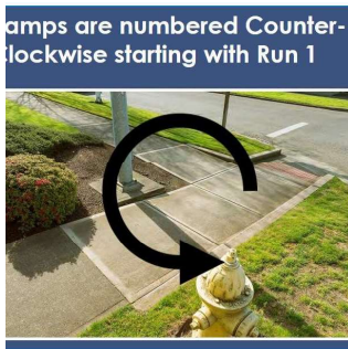
Combination Curb Ramp Numbering Scheme
