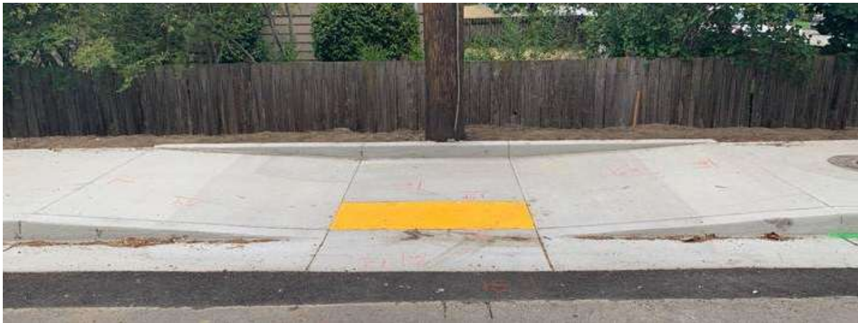
A Parallel Curb Ramp
