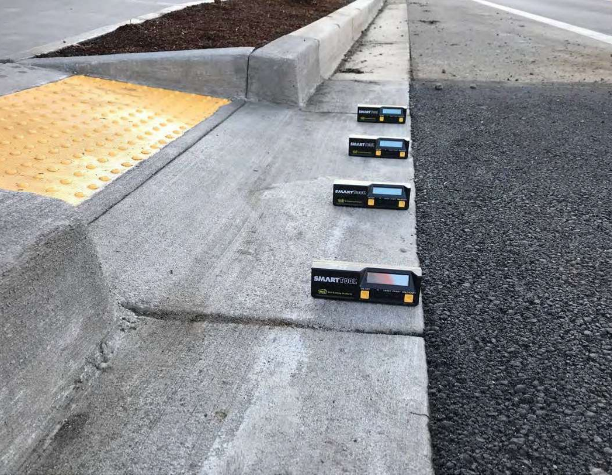
Measuring Counter Slope with a 6-inch Smart Level
