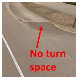
End of Walk Curb Ramp that Does Not
