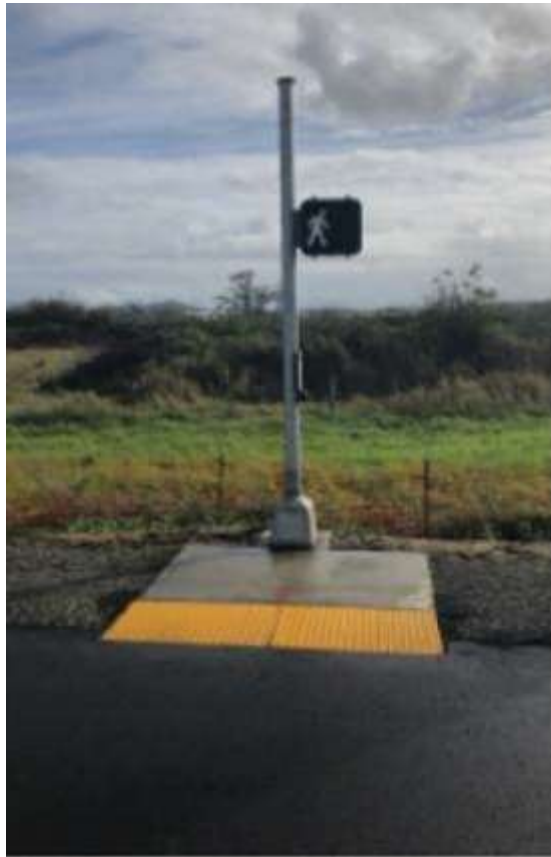
Concrete Pedestrian Pad to Access Pushbutton
