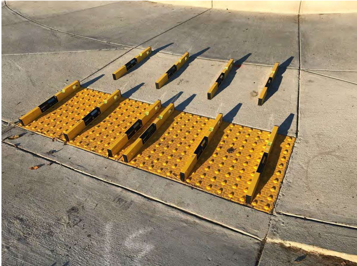
Measuring Running Slope on Ramp Run 1 On a Perpendicular Curb Ramp
