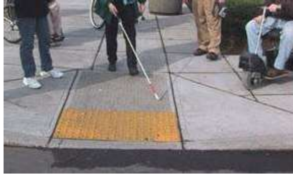
Perpendicular Style Ramp with Safety Yellow Truncated Dome Installation
