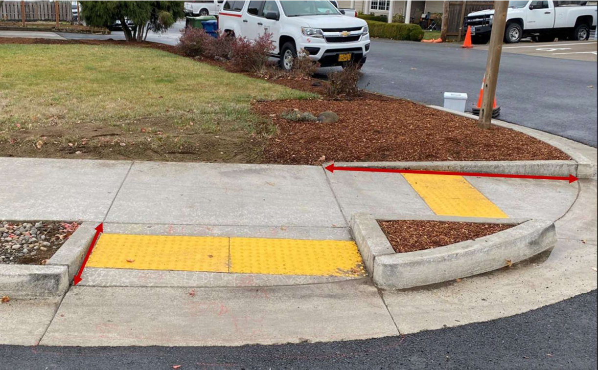
Photo of Curb Ramp System with Dimension Lines for Ramp Run Lengths.
