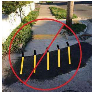
Incorrect Placement of Smart Level for Measuring Running Slope of New Asphalt Connection
