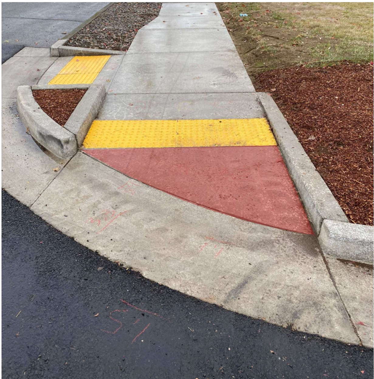
A Directional Curb Highlighted in Red
