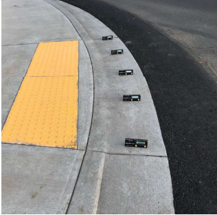
Measuring Counter Slope with a 6-inch Level
