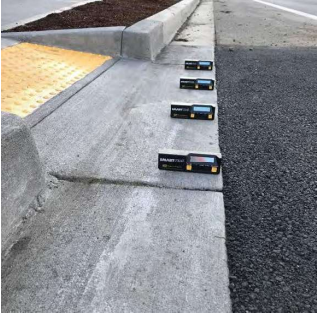
Measuring Counter Slope with a 6-inch Level
