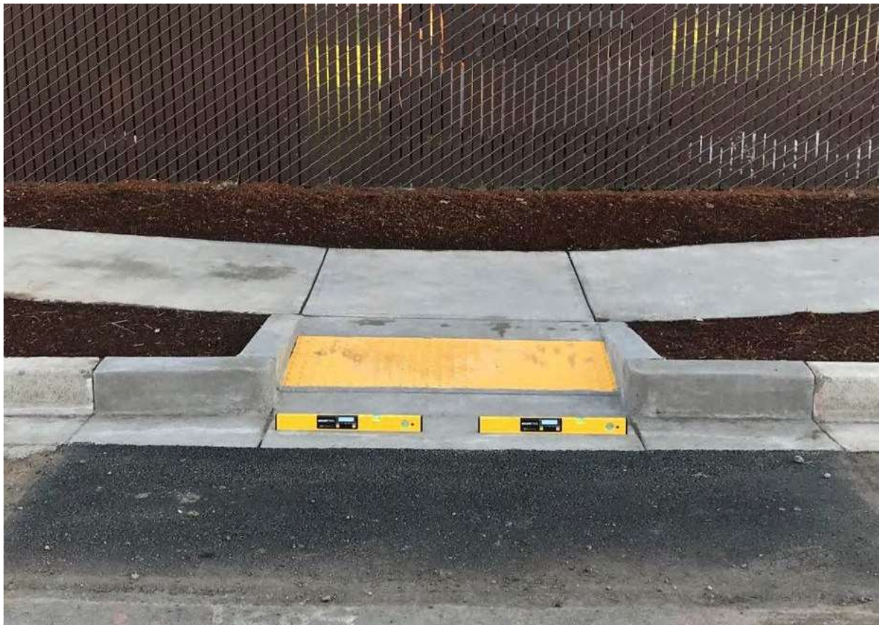
Using a Smart Level to Measure Gutter Flow Slope
