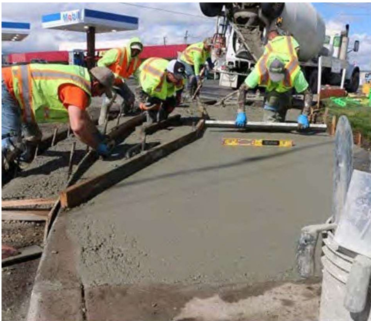
Contractor to Verify Concrete Forms
