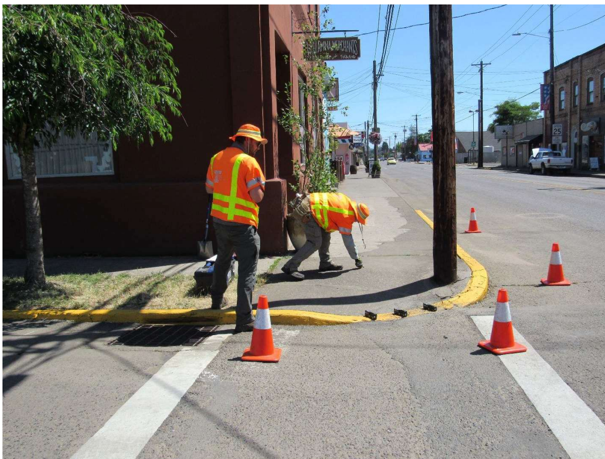
Using Traffic Cones During Inspection
