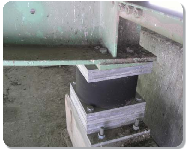
Figure 6.2 : Abernathy Bridge – Bearing Retrofit
