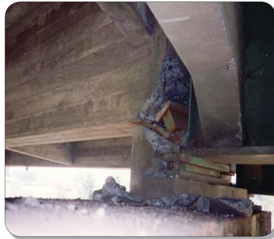
Figure 3.3: Failed Rocker Bearings (Yamhill River Bridge)
