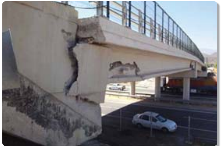
Figure B11: Shear Keys restrain the superstructure transversally during an earthquake, preventing damage
