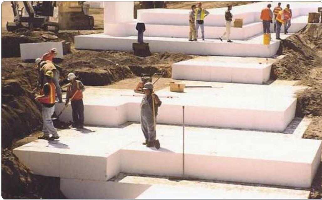
Figure B20: Lightweight fill is similar in principle to unloading: the mass of soil or rock driving the landslide is reduced by replacing it with a lightweight material such as wood chips. This method is used instead of unloading where the roadway cannot accommodate changes to the vertical alignment. The embankment is reconstructed from materials with a much lower unit weight to reduce the driving forces. Instead of having an embankment made of soil that ranges from about 95 lbs/ft 3 to 115 lbs/ft 3 , one can be constructed from material that weighs 30 lbs/ft 3 to 35 lbs/ft 3 —or about 1/3 the mass of the original embankment. An emerging technology that uses foam blocks to construct embankments is being considered. These materials weigh about 1 lb/ft 3 , which would almost negate the mass of an embankment over a landslide. In all cases, a thin layer of soil must be used to encapsulate the lightweight materials to prevent degradation that would result in excessive settlement below the road grade.
