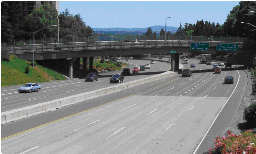
Figure B5: SW 4th Avenue over Interstate 405. Overpasses such as this may collapse during a large earthquake and will be difficult to repair or replace without further disruption of I-5 traffic.
