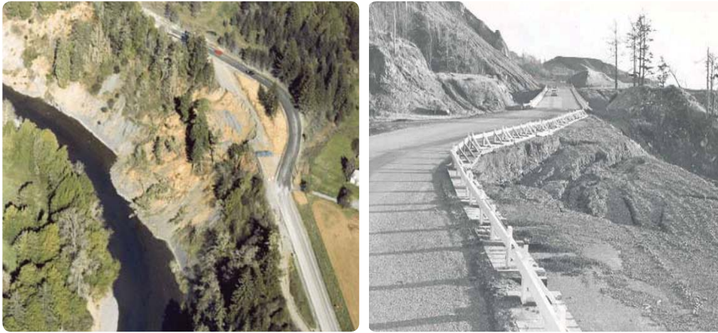
Figure B7: Two examples of temporary slide bypasses
