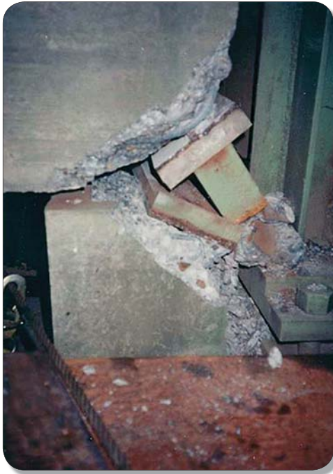
Figure D4: Failed Rocker Bearings (Yamhill River Bridge)
