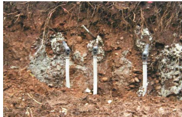
Figure B19: Drainage is one of the most cost-effective methods of landslide mitigation and usually forms some aspect of every landslide mitigation design. Water increases the weight of a slide mass while decreasing the shear resistance of soil and rock materials, so removing it greatly improves stability. One method is to construct trench drains, a feature commonly known as a French drain. Trench drains are used to intercept subsurface water and conduct it to nearby streams or storm drain systems. The drain can be dug as deep as an excavator can reach, sometimes up to 20 feet deep. Gravel backfill intercepts the groundwater and allows it to seep down to the perforated pipe. From there, it flows to the intended location away from the landslide. Horizontal drains are used to remove groundwater from deep within a slide mass. They are constructed by drilling holes horizontally into the slide and past the slide surface. Pipes with slotted sections to allow inflow are inserted into the drill holes and sealed at the surface with cement grout to prevent erosion at the pipe outlet. Horizontal drains are targeted at water-bearing zones identified by exploratory drilling during project design. A drainage-only approach to slide mitigation will not eliminate slide movement. It will, however, reduce the rate of movement of the largest landslides to manageable levels. Effective slide drainage also improves performance during a seismic event, as less water in the slide mass improves its reaction to strong ground shaking and reduces the effects of liquefaction.
