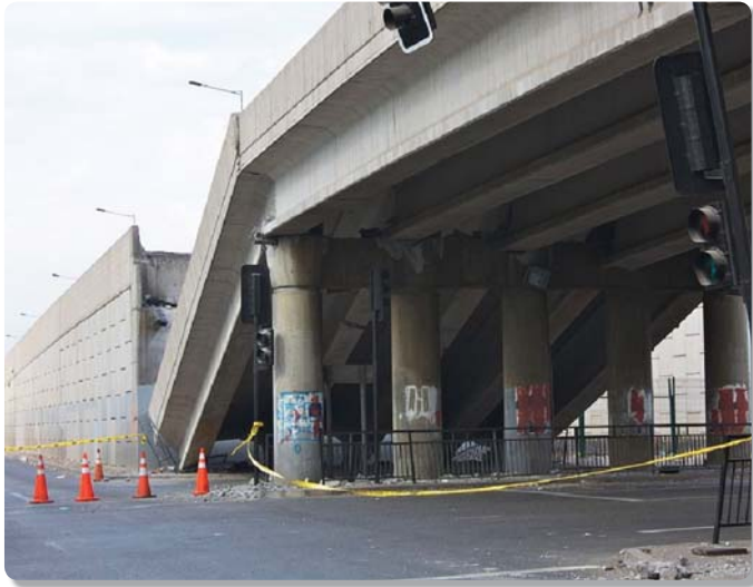
Figure B10: Restrainer Cables will prevent the bridge superstructure fall-off
