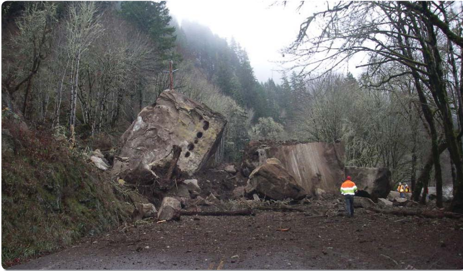
Figure B6: Hwy38 Rockfall site not previously known to be unstable
