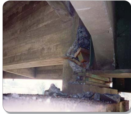
Figure D4: Failed Rocker Bearings (Yamhill River Bridge)
