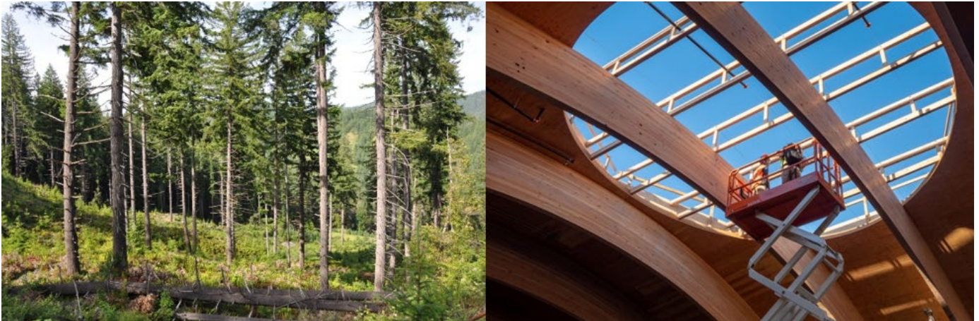
The Glulam beams for the wooden roof in PDX’s new terminal were sourced from the FSC-certified Coquille Tribal Forest. Source: USDA, Oregon NRCS (left), PDXNext (right)
