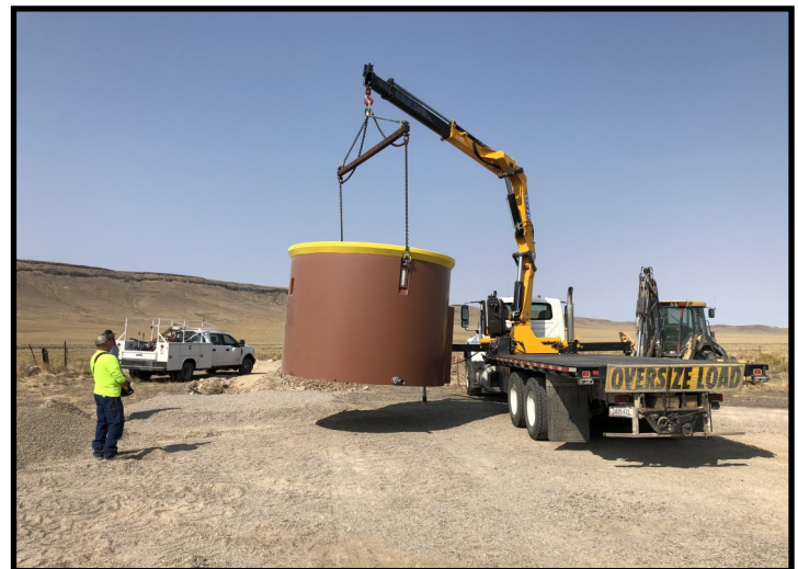
Blue Mountain RFPA and Vale BLM installing the new heli-well
