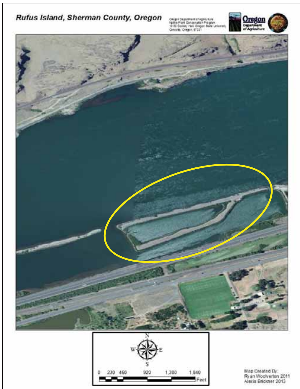
Figure 3.1. Rufus Island (see yellow circle). is located approximately 5 miles west of the town of Rufus, OR. It is part of a series of cobble bars created during dam construction. Interstate-84 runs adjacent to the island.
